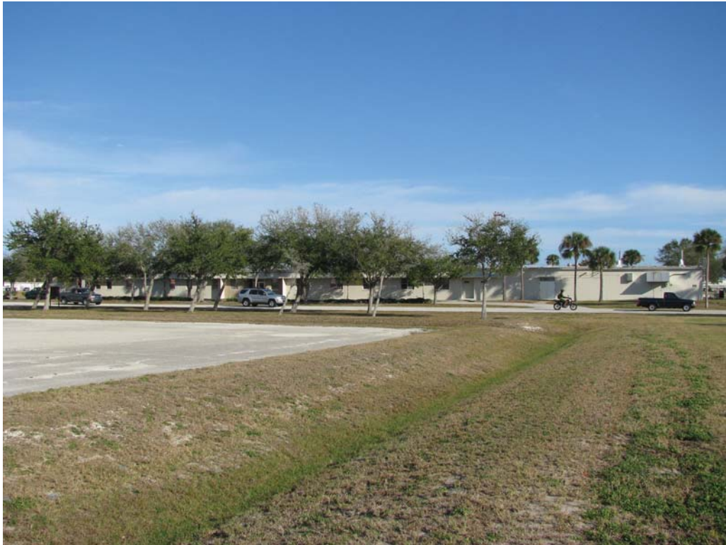
West elevation, facing east
