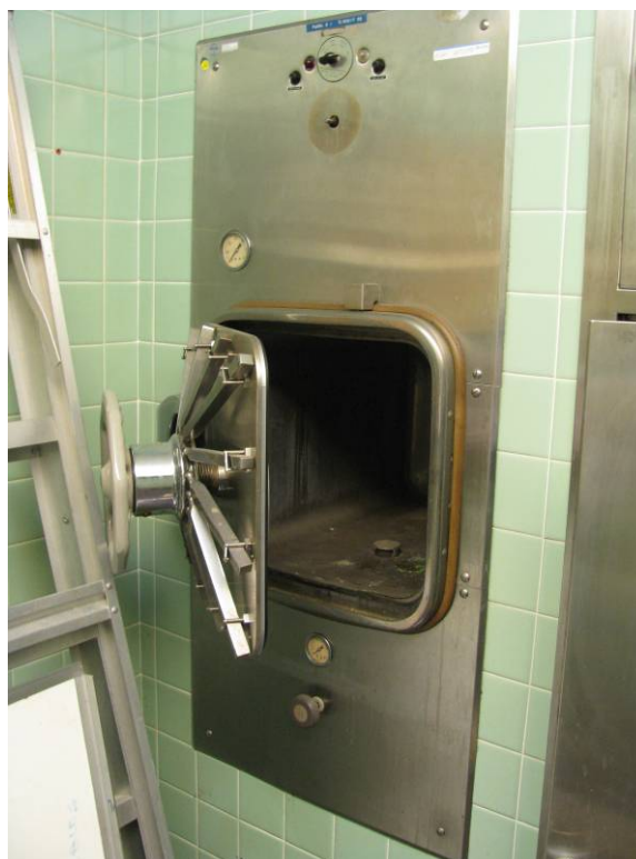
Photo 13. Detail of the original sterilizer, facing northeast.
