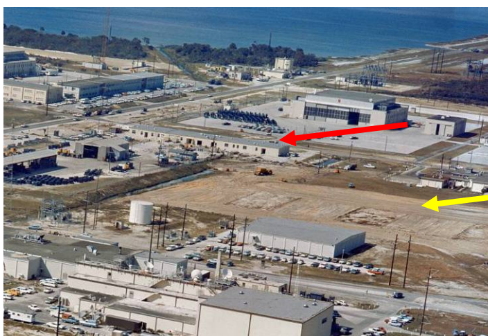
Photo 8. BOSU (red arrow) under construction ca. 1964, facing southwest. Yellow arrow denotes heliport. (Kennedy Institutional Imaging Facility, PL64C-82448).
