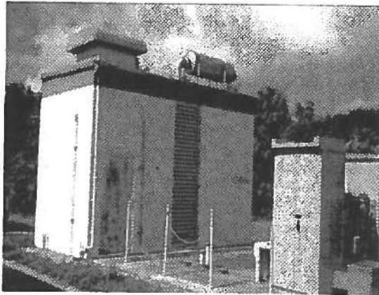
K7-1557A – Generator Building - Built in 1965 – Service Building - Launch complex building housing equipment; mothballed in 1995.
