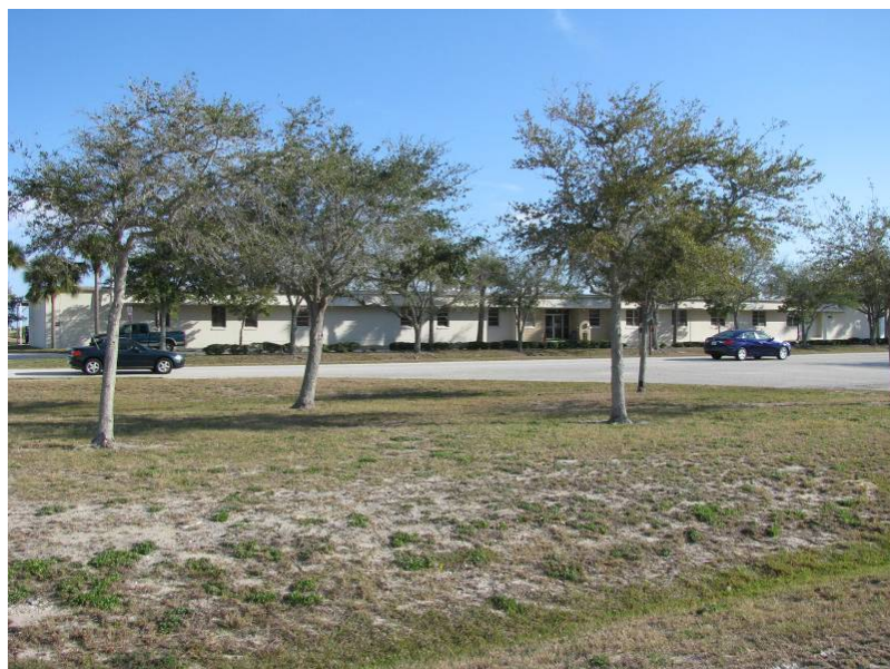
Photo 11. West elevation of the BOSU, facing southeast.
