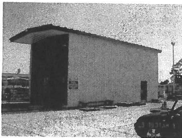
M6-0536A – POL – Built in 1996 - Flammables Storehouse- Facility used for storage of inflammable and combustible material (includes paints, POL products, oils, etc.).
