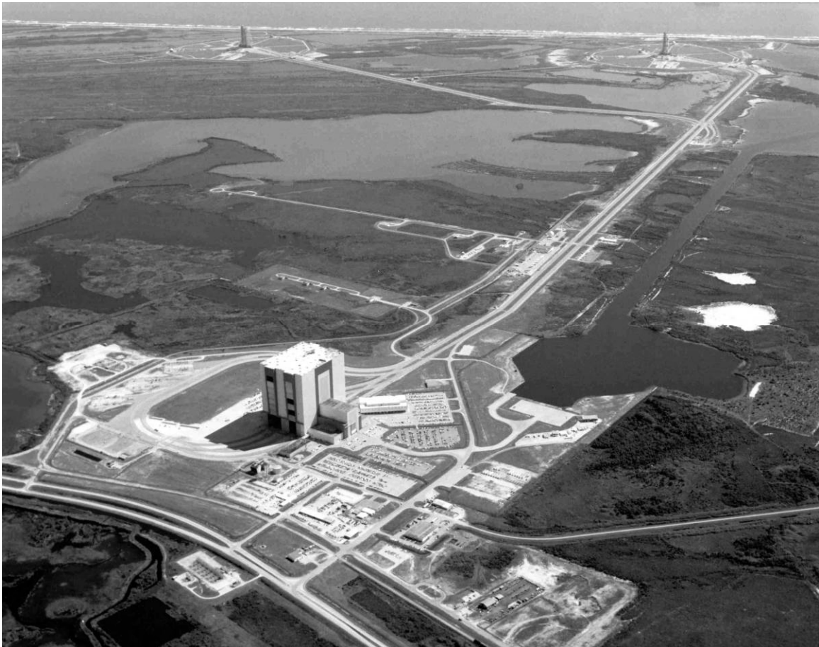
Figure A-1. Aerial view of Launch Complex 39 showing the Crawlerway, camera facing northeast, April 16, 1973.
