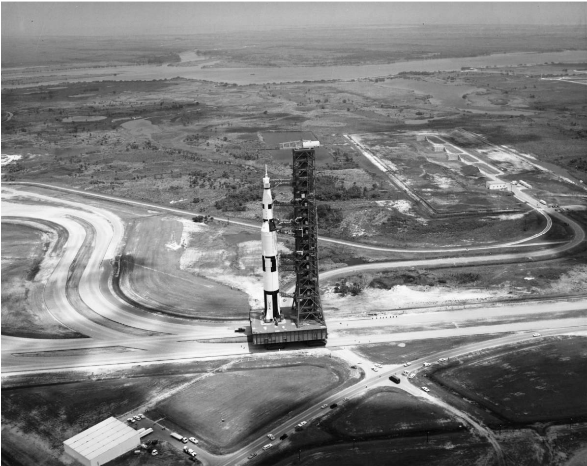
Figure A-9. Crawlerway in use as crawler transporter carries the Apollo 500-F test vehicle to LC 39A, May 25, 1966.
