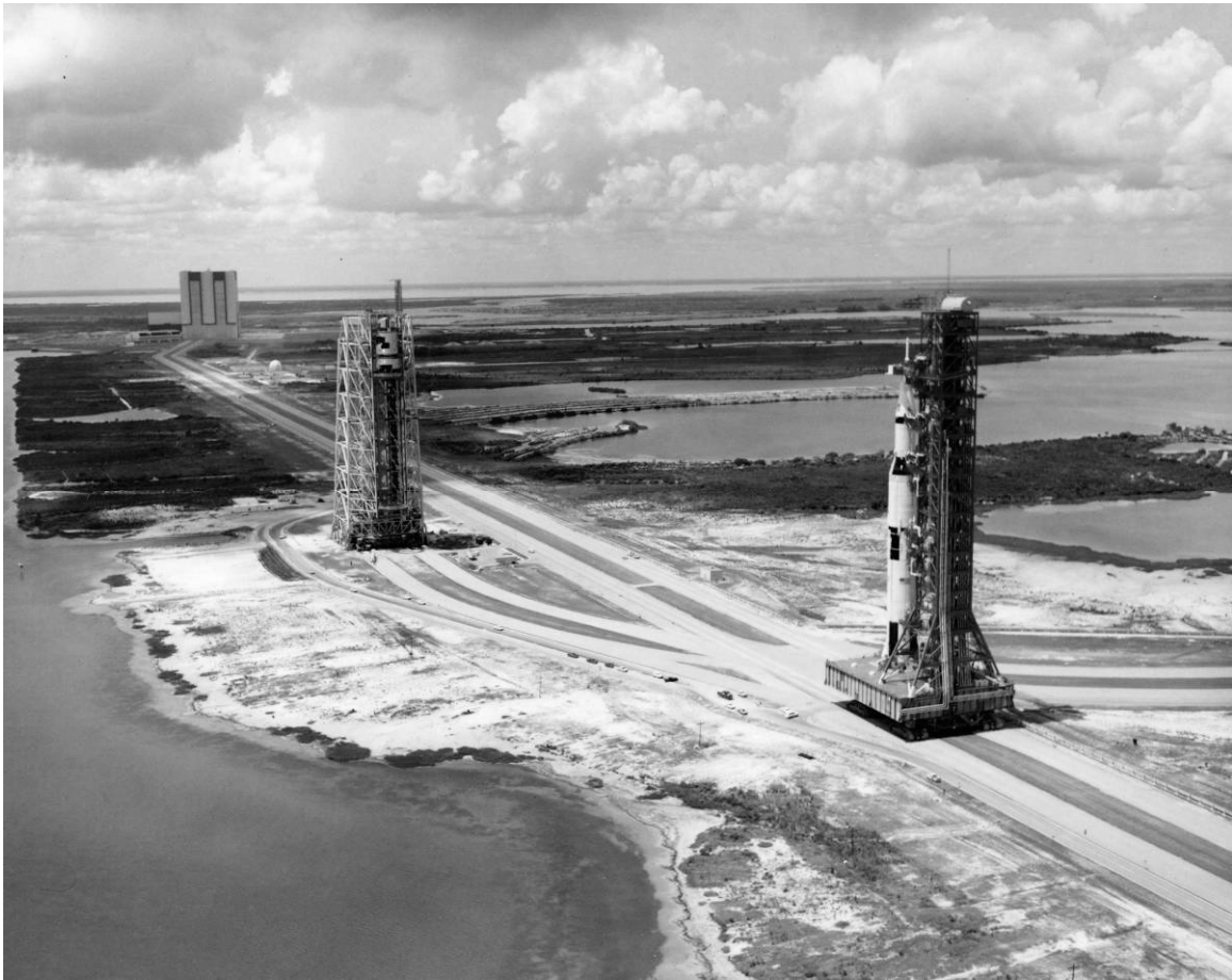
Figure A-10. Crawlerway in use as crawler transporter carries Apollo 4 to LC 39A, August 26, 1967.
