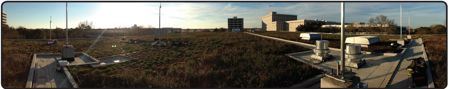
JSC Building 12 Green Roof with Wind and Water Instrumentation
