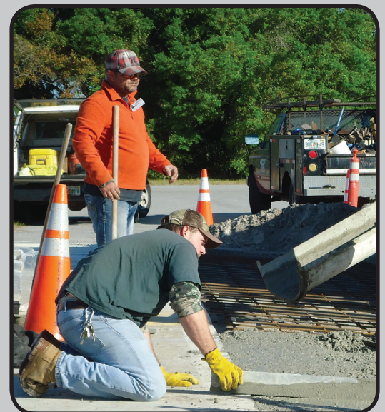
Laying Concrete with SBM as an Aggregate at KSC
