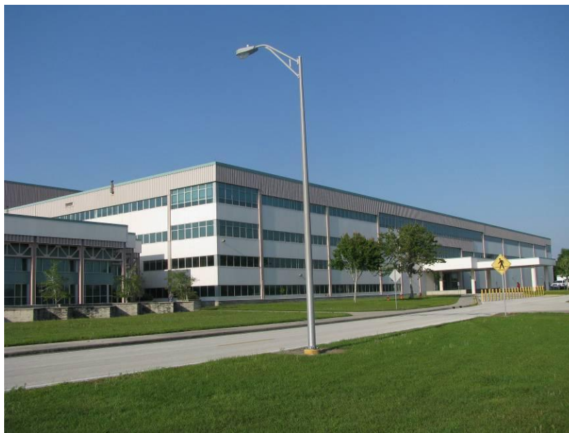
Photo 13. North and partial east elevations of SSPF, facing southwest. (Archaeological Consultants, Inc., 2010).
