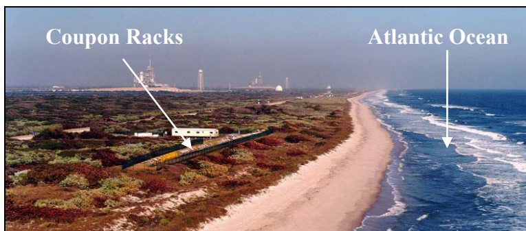
Figure 4-14 Beach Corrosion Test Site at KSC
