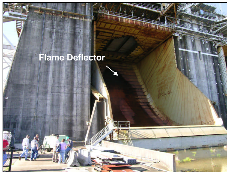
Figure 5-1 Stennis Space Center Rocket Motor Test Stand
