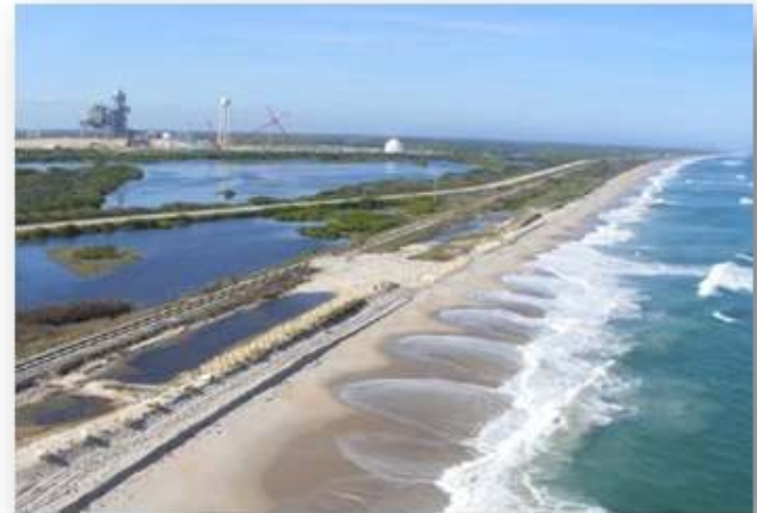
View of KSC after heavy rain event
