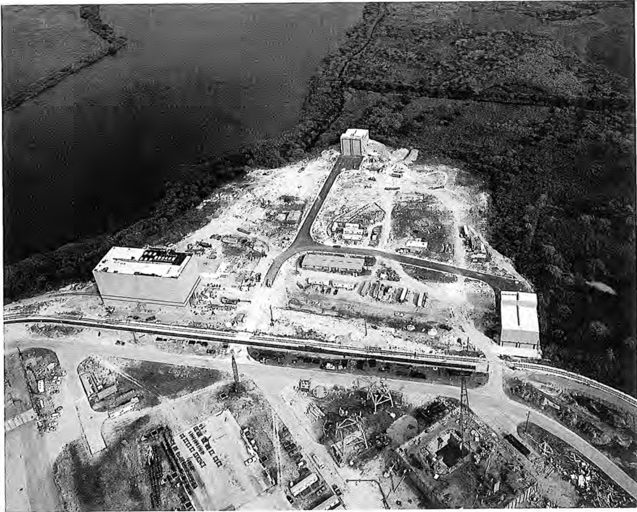
Aerial View of RPSF Complex Under Construction, View to North, October 4, 1983 (Courtesy of Kennedy Space Center, Negative 116- KSC-383C-3563-20).
