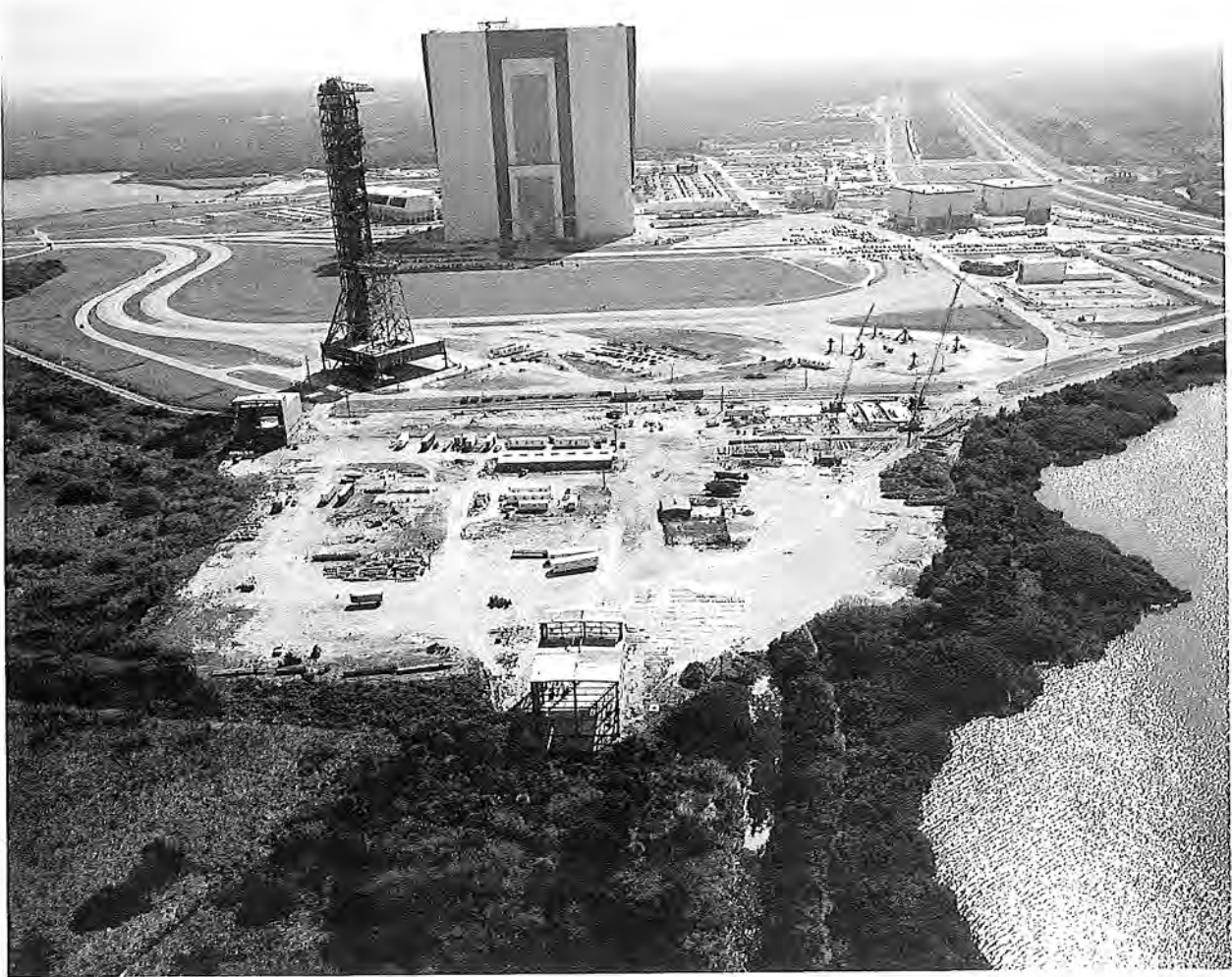
Aerial View of RPSF Complex Under Construction at Bottom of Photograph, View to South, February 8, 1983 (Courtesy of Kennedy Space Center, Negative 108-KSC-383C-267-20).
