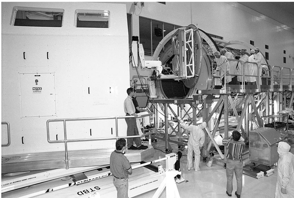
Figure A-17. Removing the end cap of the Multi-Purpose Logistics Module, Leonardo , using the Rack Insertion Device, camera facing southwest, August 4, 1998.
