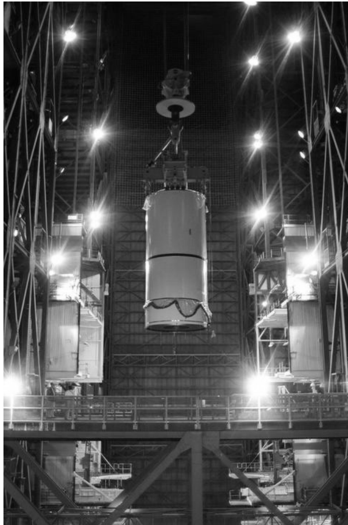
Photo A-9. A SRB segment being lifted over 192' level for stacking, 30 November 2004. Source: John F. Kennedy Space Center, KSC-04PD-2420, via http://mediaarchive.ksc.nasa.gov/search.cfm .
