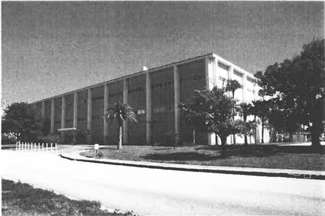
Central Instrumentation Facility, north and west elevations, facing southeast
