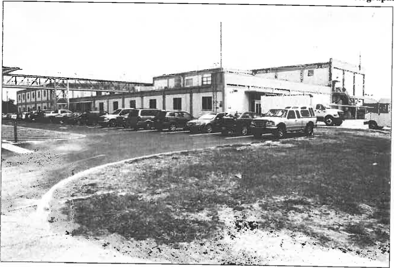
Engineering Development Laboratory (M7-0409) Exterior Oblique, View Southeast
