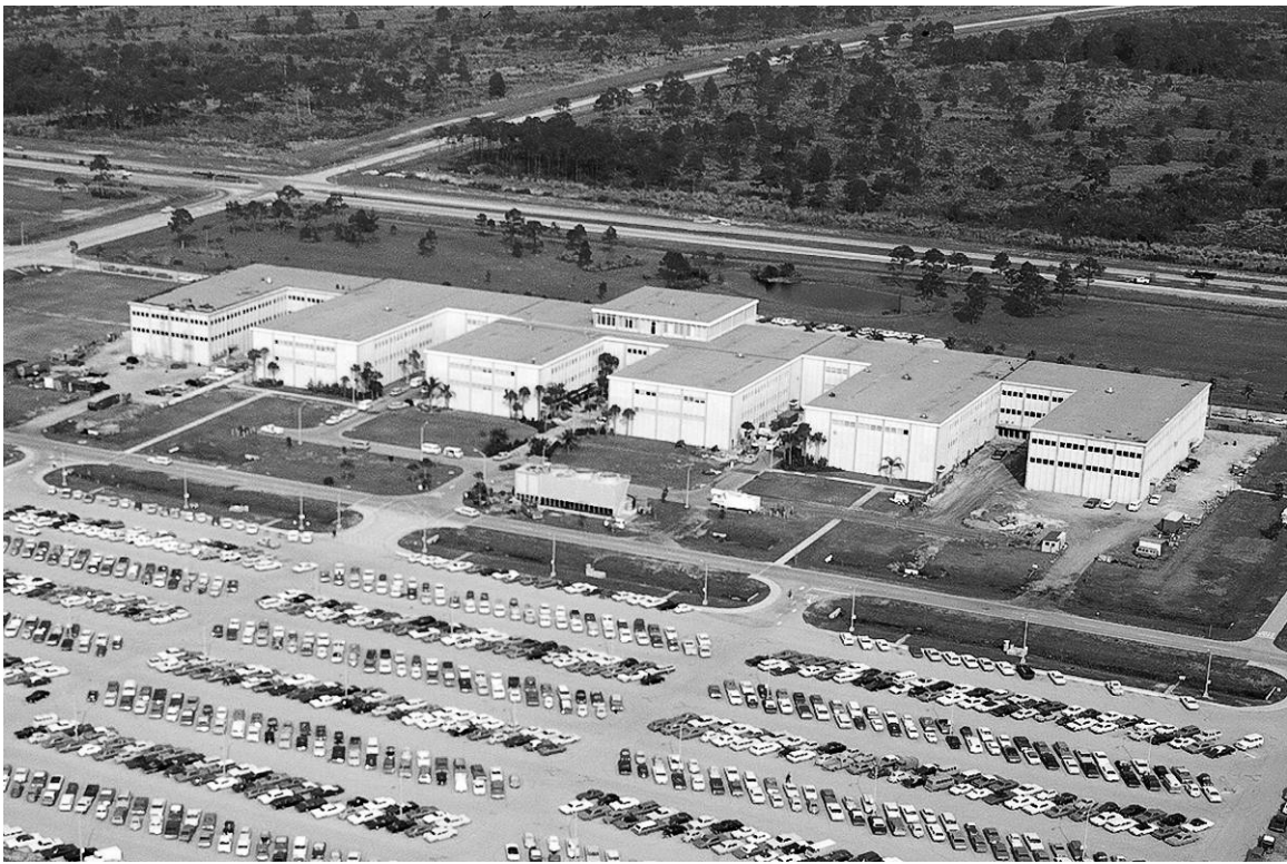
Figure A-15. Aerial view showing near completion of east and west wings, facing northwest, January 10, 1968.
