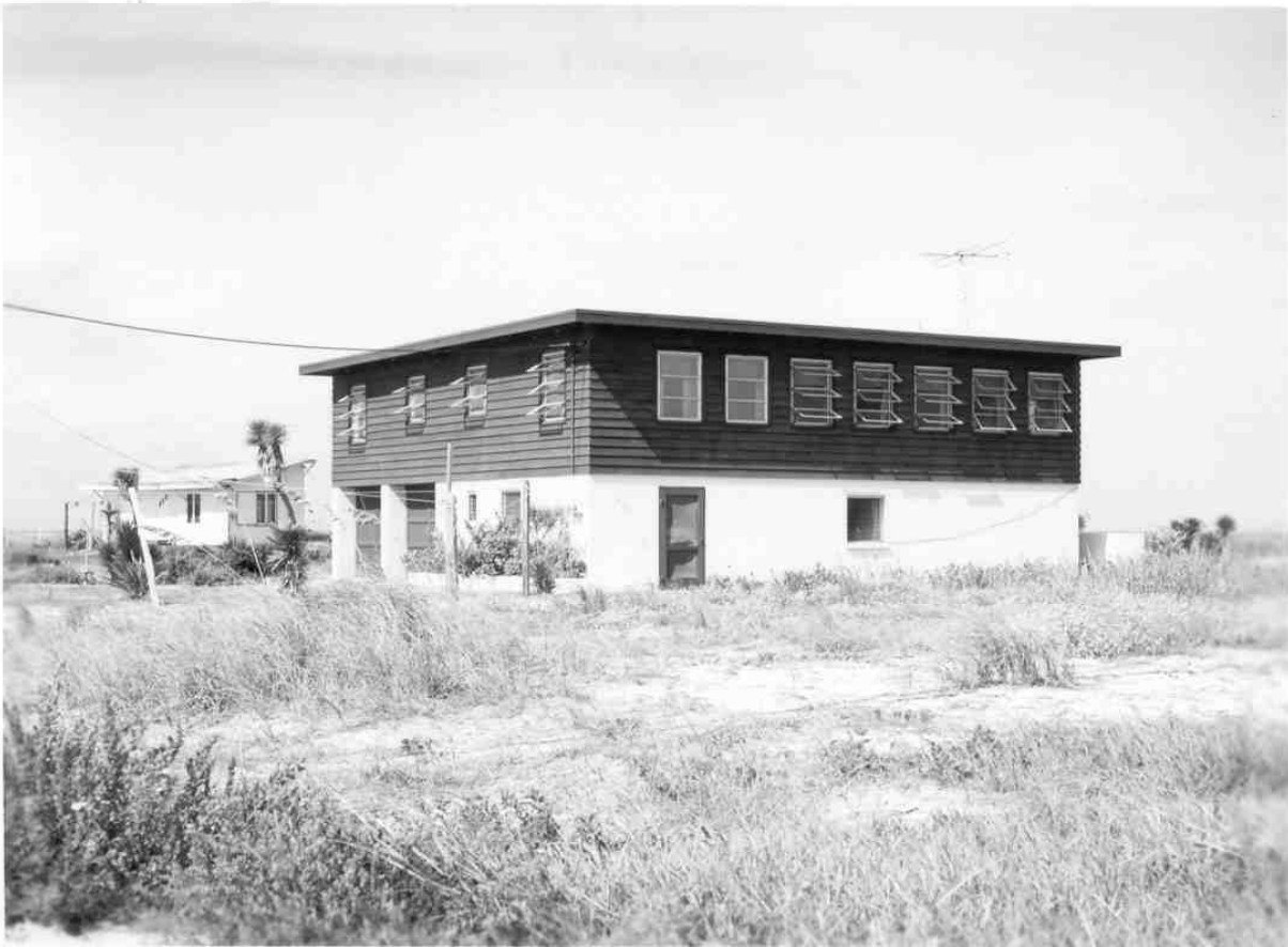
Figure 5. Circa 1963 photograph of the Beach House with another house in the background before it was demolished by NASA KSC. Note the original awning windows of the Beach House are open. Oblique view to the northeast. (Courtesy of Kennedy Space Center Archives, no negative number).
