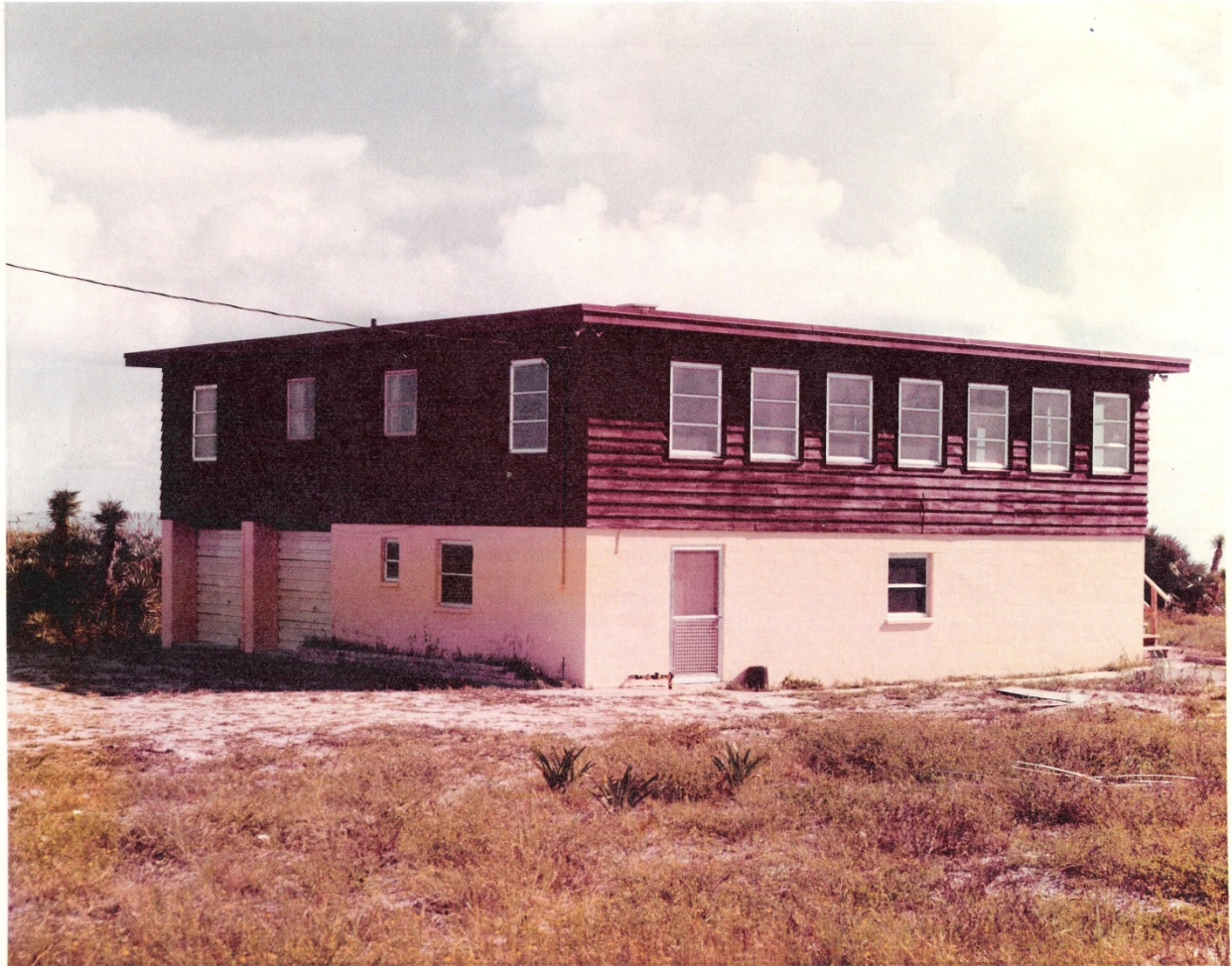
Figure 7. 1974 photograph of the Beach House, oblique view of the west (rear) and south elevations, view to the northeast. (Courtesy of Kennedy Space Center Archives, Image 116-KSC-74C-940).
