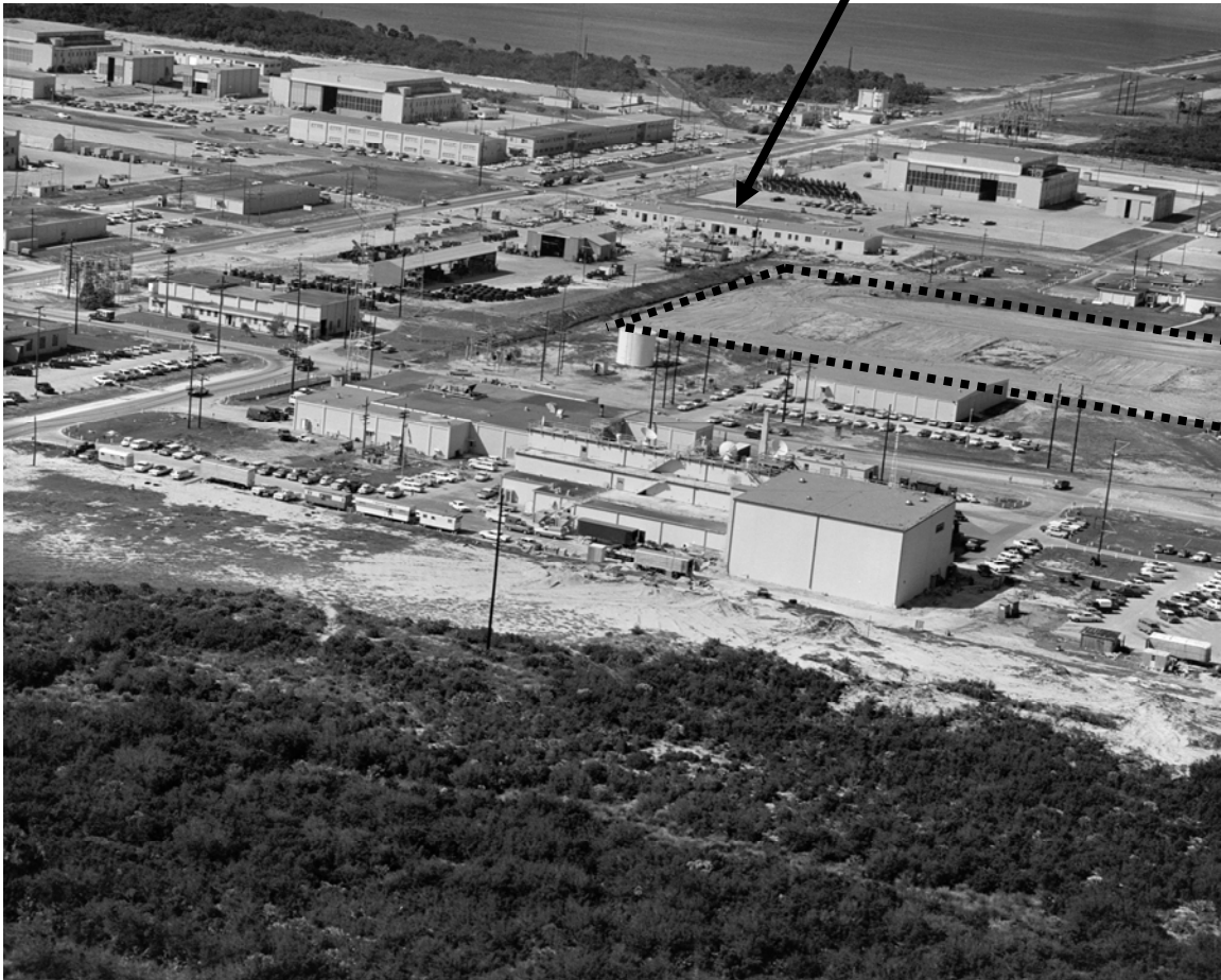
Figure A-1. BOSU (denoted by arrow) under construction circa 1964; the heliport is denoted by the dashed lines. Source: John F. Kennedy Space Center, Kennedy Institutional Imaging Facility, PL64C-82448.
