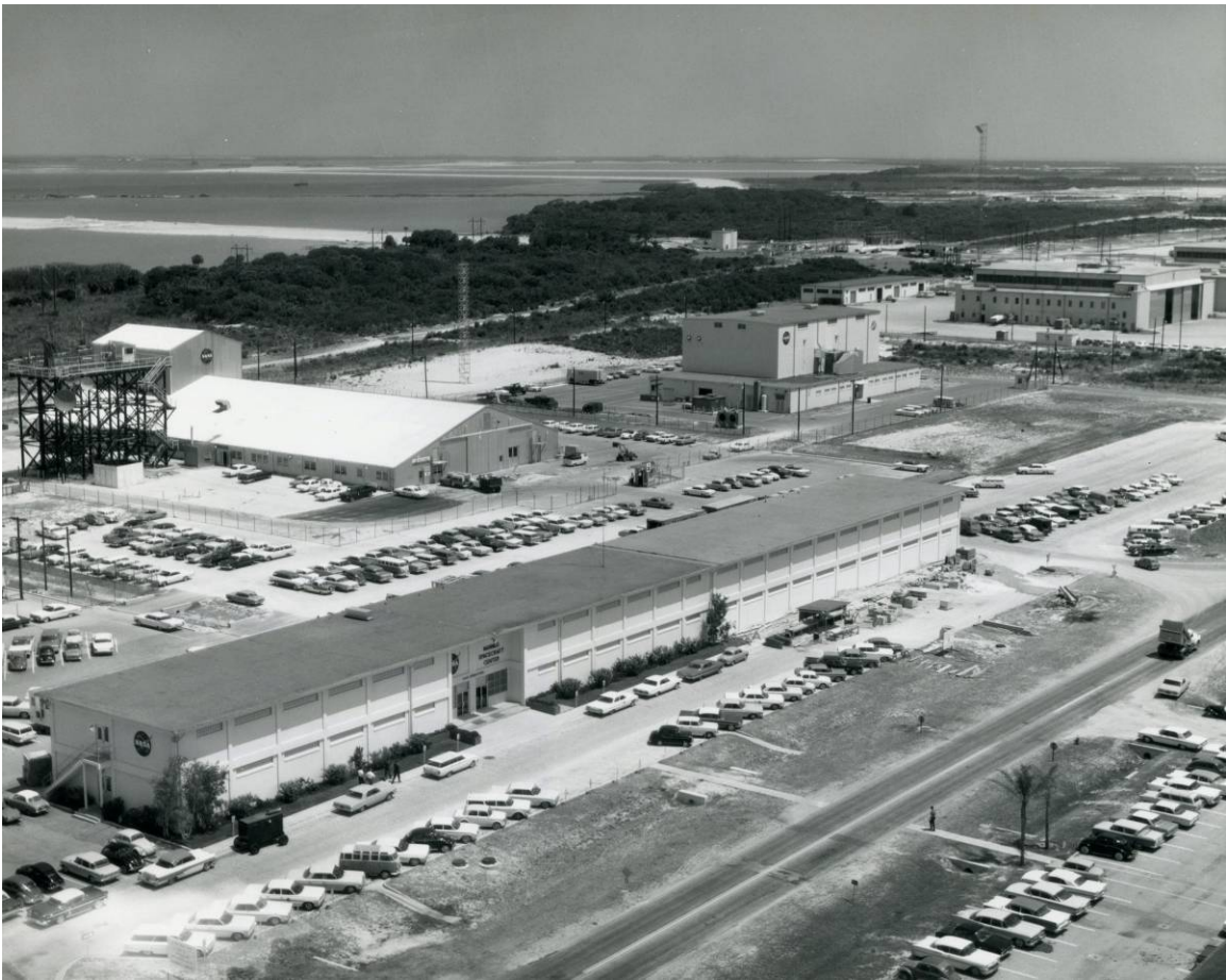
Figure A-6. View of E&O Building with completed North Wing addition, May 17, 1963. Source: John F. Kennedy Space Center Archives, LOC-63-4892.
