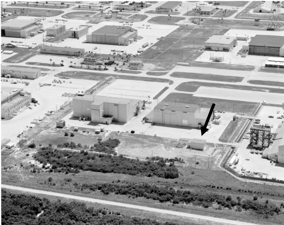
Figure A-3. Aerial photograph with Solar Array Test Building (denoted by arrow), April 17, 1973.
