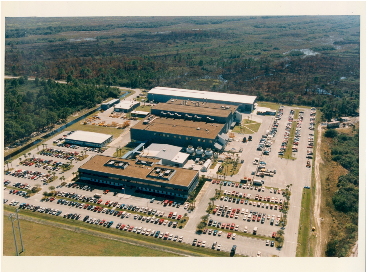
Aerial Photograph of the SRB ARF Manufacturing Building, View Southeast, 1996. (Courtesy KSC, Image KSC-396C-0968.36).
