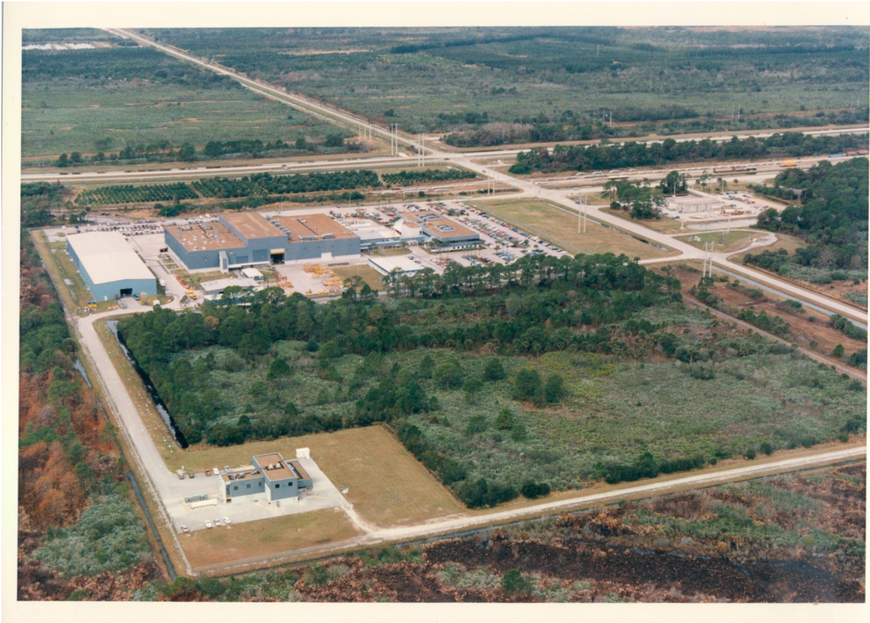
Aerial Photograph of the SRB ARF Manufacturing Building, View Northwest, 1996. (Courtesy KSC, Image KSC-96PC-209).
