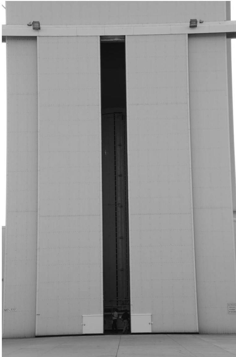
Figure A-21. Detail view showing the CRF doors opening, April 15, 2010. Source: Penny Rogo Bailes.
