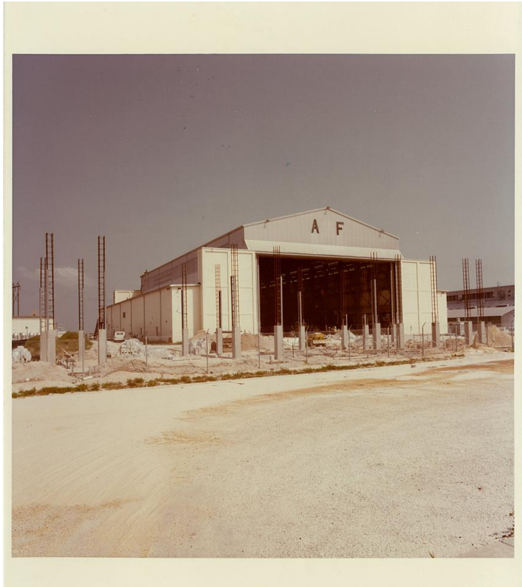
Figure 9. Construction of the First Wash Building and SRB dolly rails with Hangar AF in the Background, 1978. (Courtesy KSC, Image 108-KSC-378C-759).
