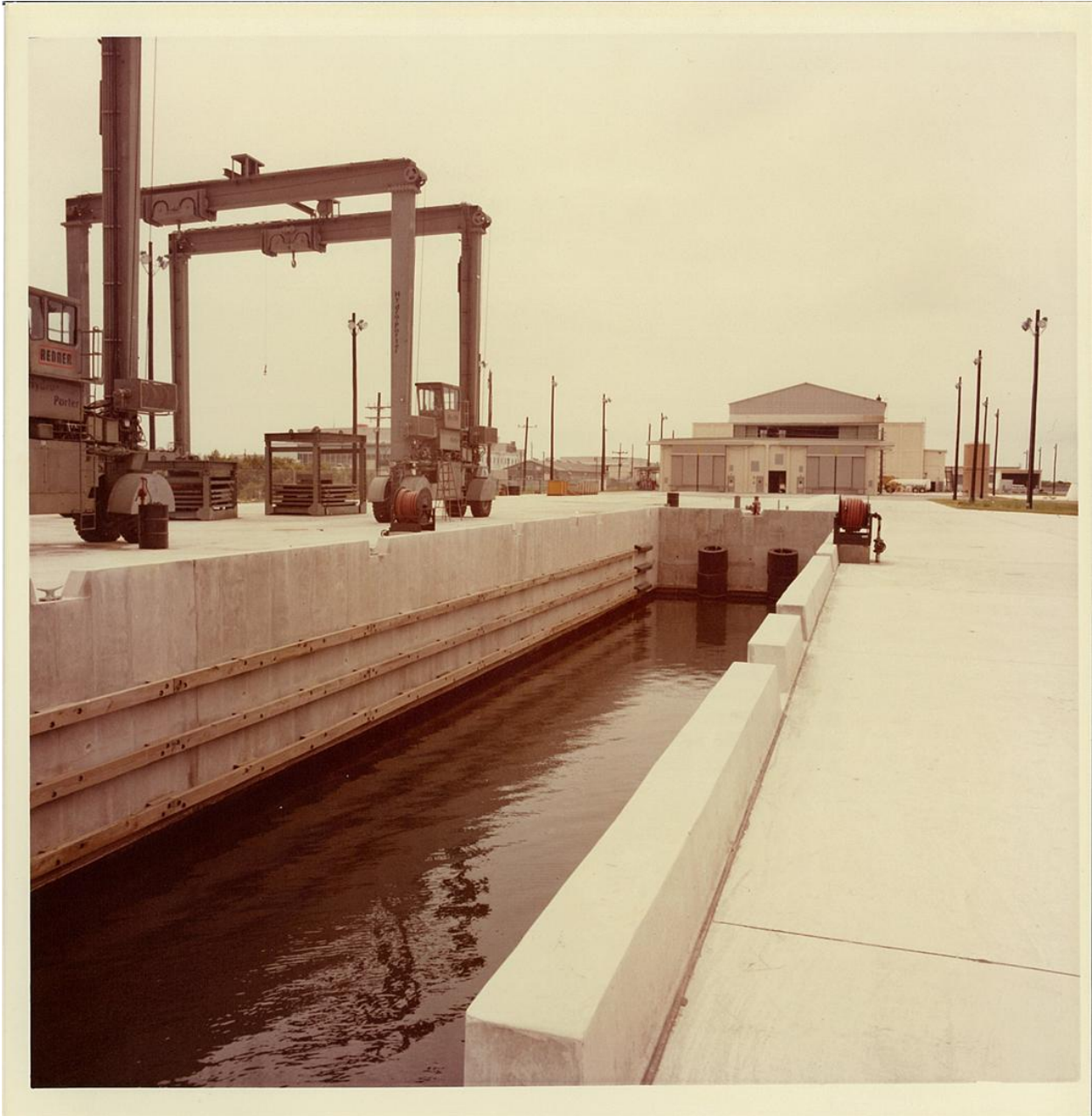
Figure 12. SRB Recovery Slip with gantry cranes, First Wash Building, and Hangar AF, 1978. (Courtesy KSC, No Image Number).
