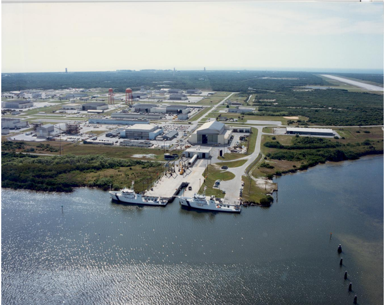
Figure 7. This 1983 aerial photograph shows the condition of the complex and its relationship to the CCAFS Industrial Area. (Courtesy of KSC, Image 116-KSC-383C-1256).
