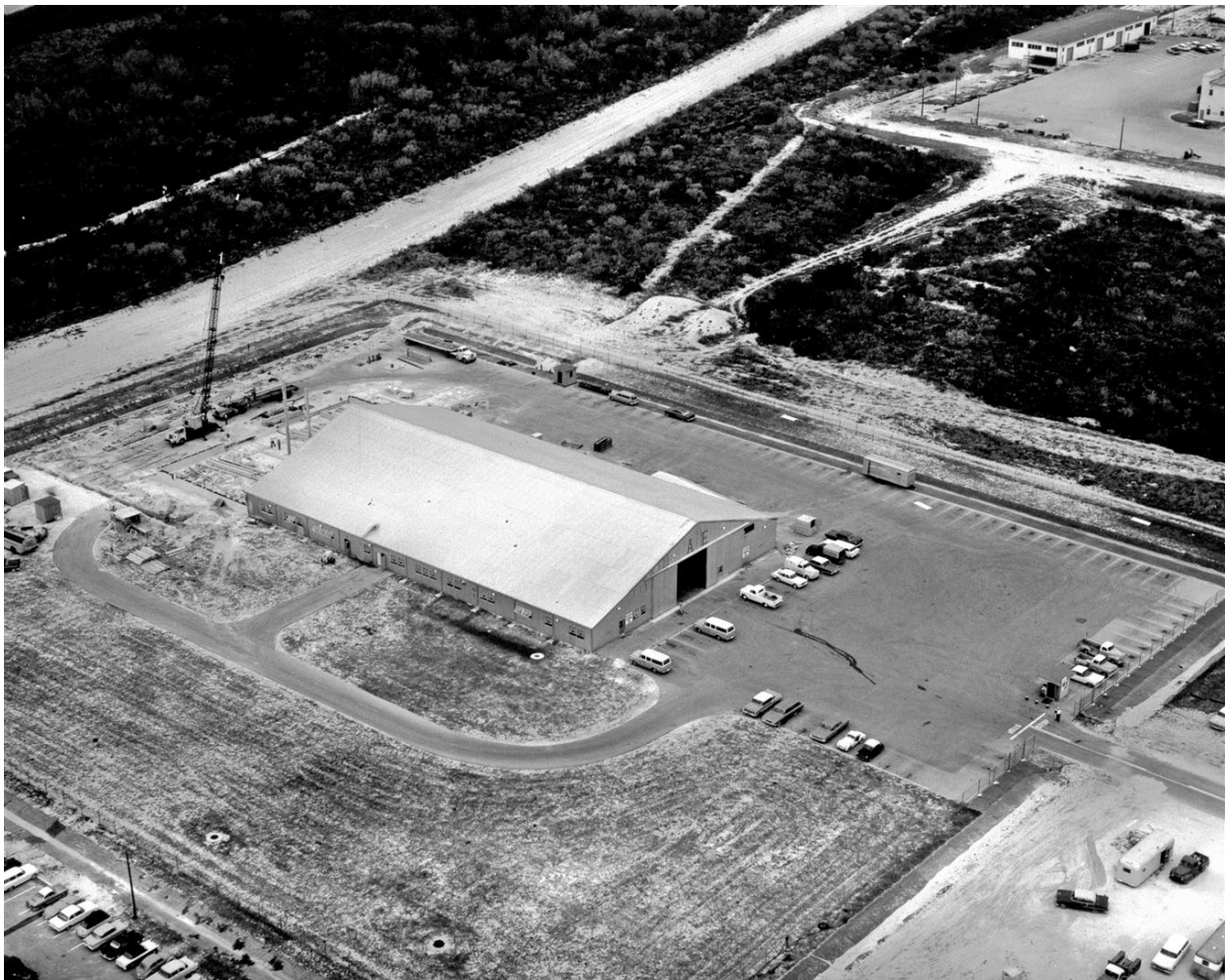
Figure 3. Aerial view of Hangar AE, 1961. (Courtesy of Kennedy Space Center Archives, Image LOD-61-2195).
