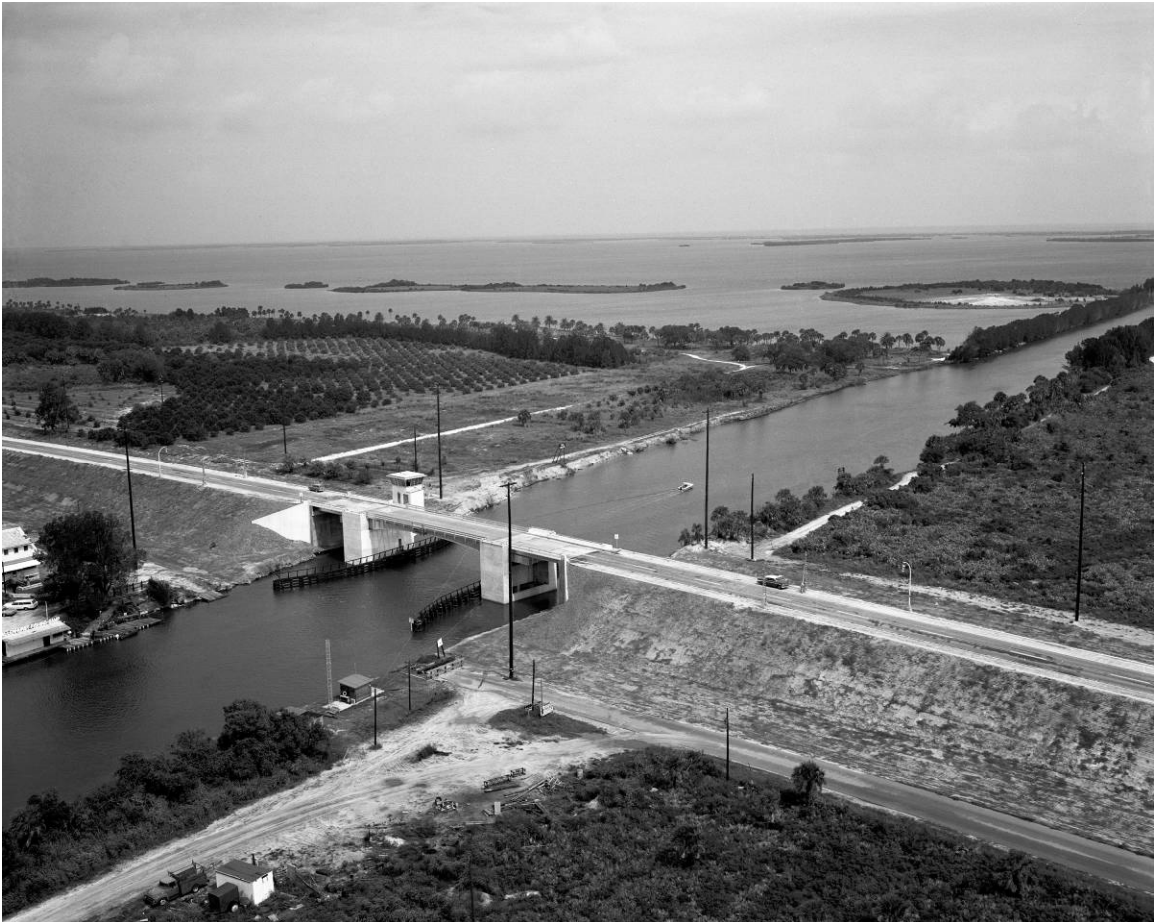
Figure A-5. Aerial of the completed Haulover Canal Bridge (following removal of old wooden bridge), camera facing north, October 5, 1965.
