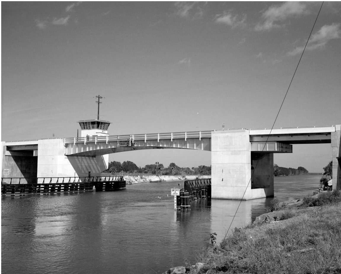
Figure A-6. Ground level view of the completed Haulover Canal Bridge, camera facing north, January 12, 1966.
