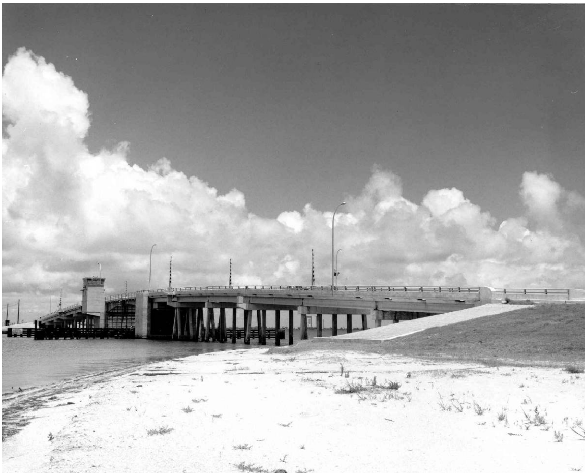
Figure B-7. Banana River Bridge, facing northwest, June 29, 1965. Source: John F. Kennedy Space Center Archives, 100-KSC-65-12643.
