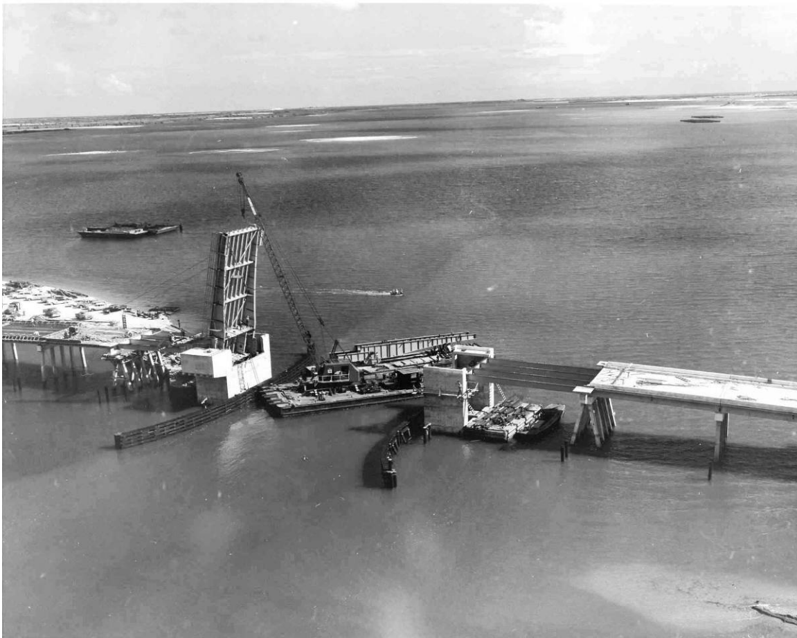
Figure B-5. Construction of the Banana River Bridge, facing northwest, September 10, 1963. Source: John F. Kennedy Space Center Archives, LOC-63-9113.
