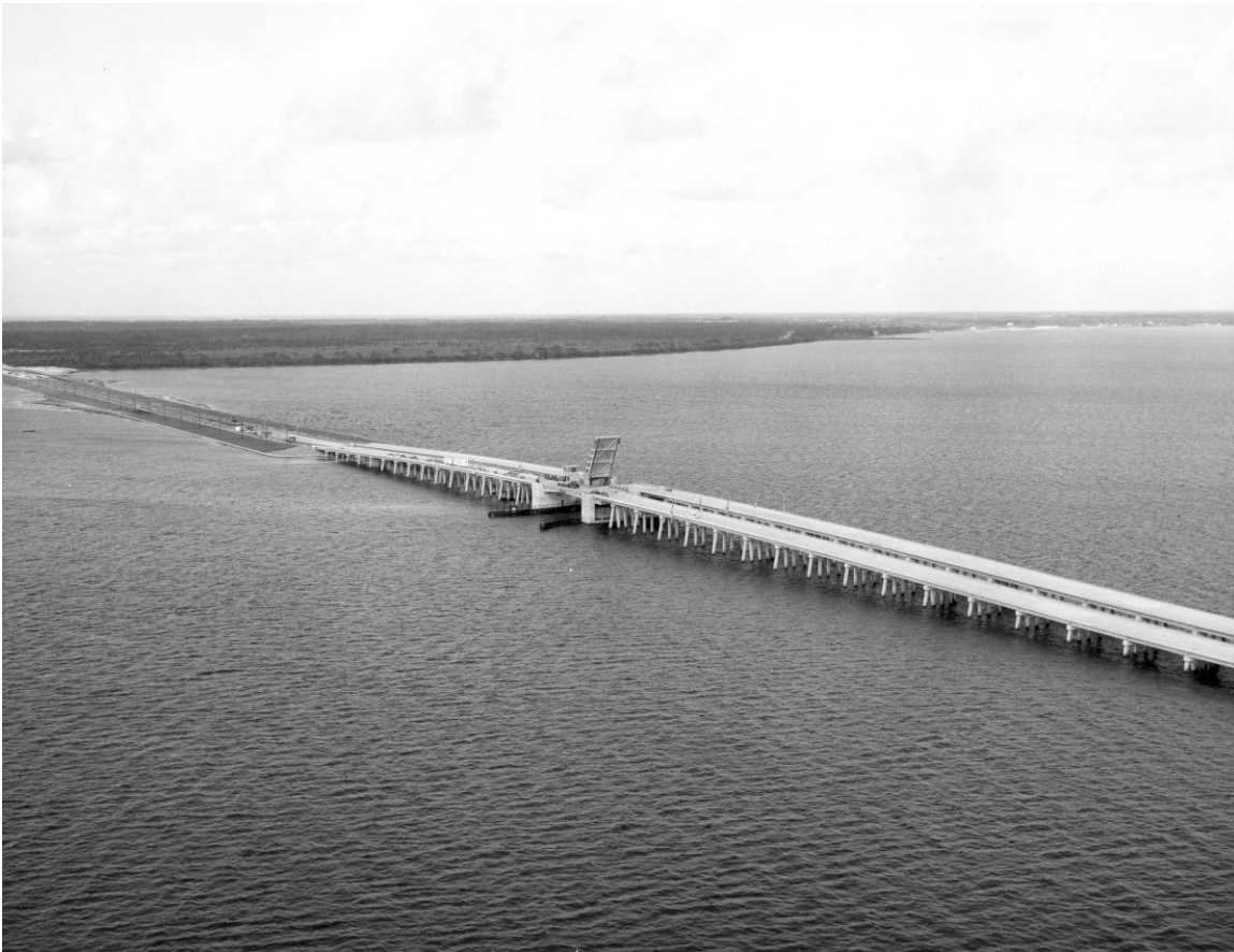
Figure B-12. Construction of the Indian River Bridge, facing northwest, October 13, 1964. Source: John F. Kennedy Space Center Archives, 100-KSC-64-18836.
