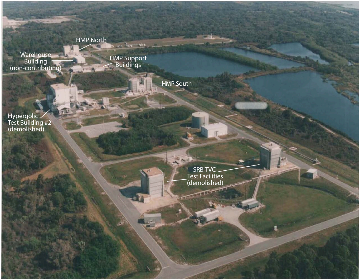
1996 aerial view to the northeast showing the HMCA complex before demolition of the SRB TVC Test Buildings and Hypergolic Test Building 2. (Courtesy KSC: Image KSC-396C-0940-10)
