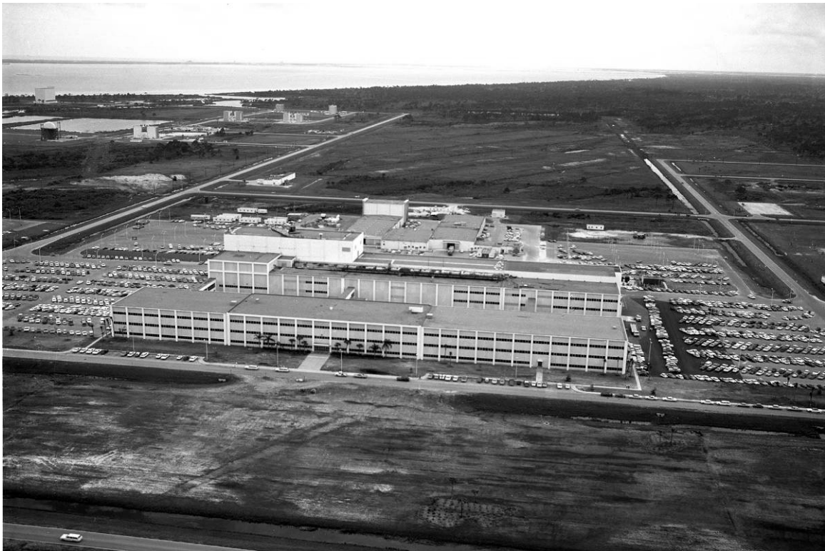
Figure B-10. Aerial of the O&C Building with the completed exterior shells of the additions, facing south, June 21, 1966.
