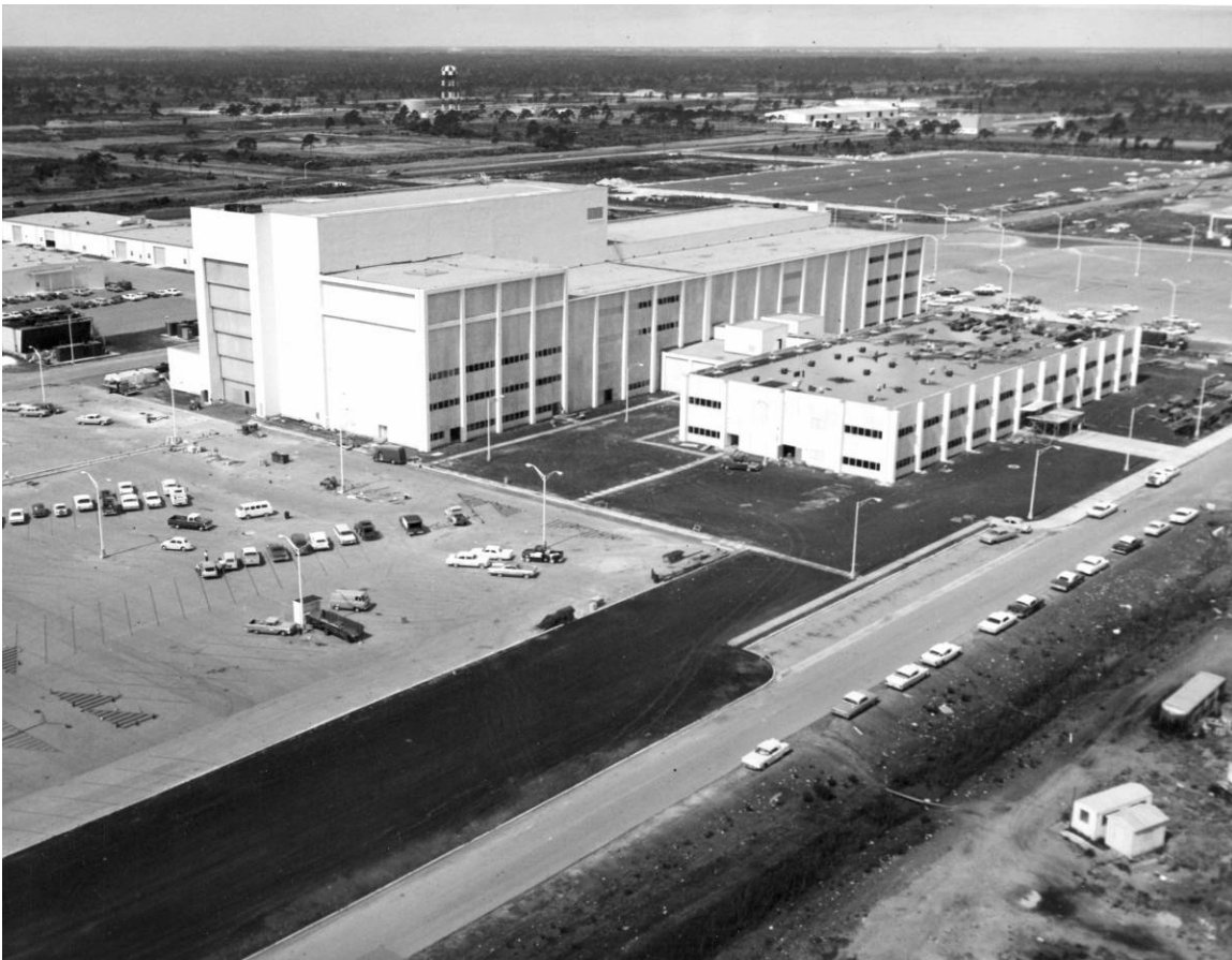
Figure B-7. Construction of the original O&C Building nearing completion, facing southwest, June 25, 1964.
