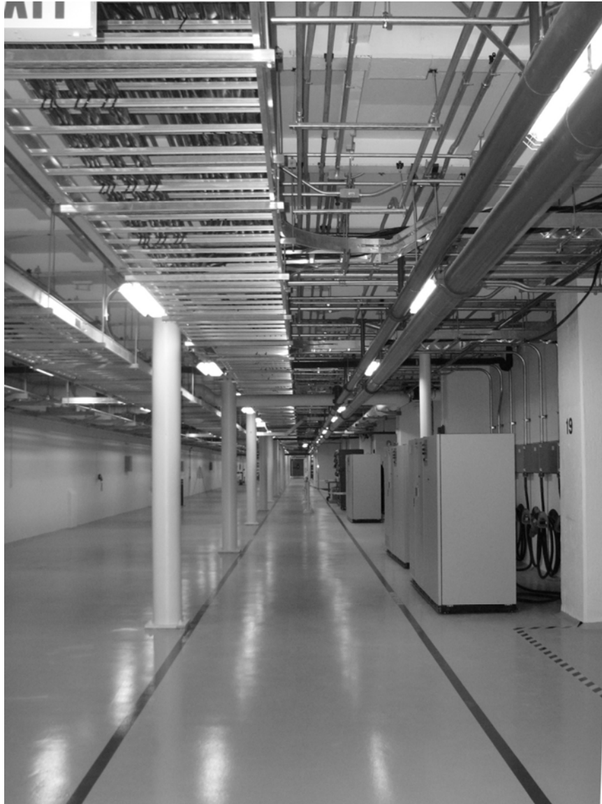
Figure B-28. View of the cable/utility tunnel, circa 2010. Source: Lockheed Martin.
