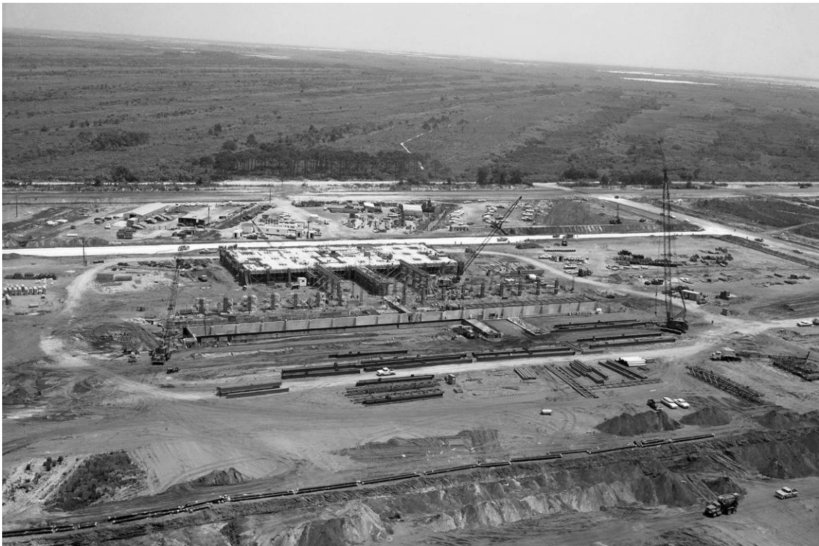
Figure B-2. Early construction of the O&C Building, facing northeast, May 17, 1963. Source: Kennedy Institutional Imaging Facility, KSC-63C-1682.
