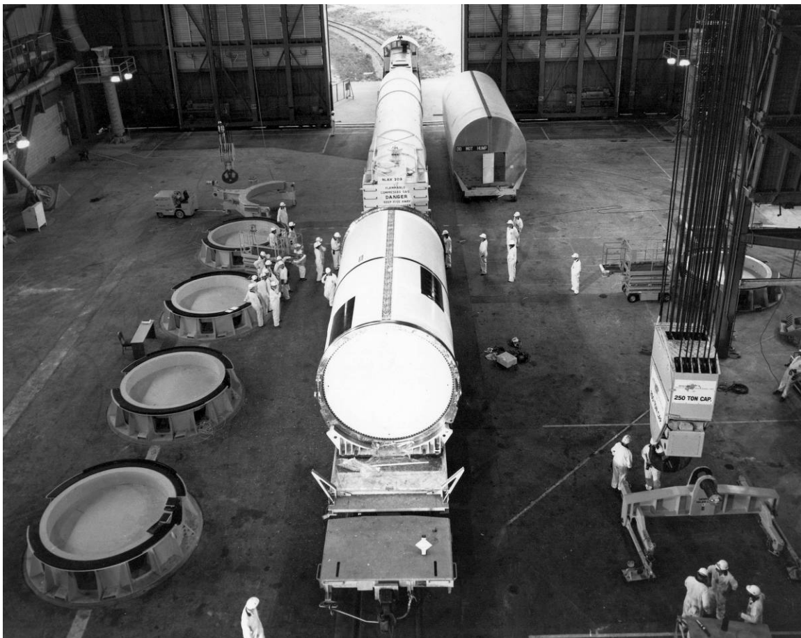
Figure A-9. Fueled SRM segments being offloaded in VAB High Bay No. 4, November 29, 1979.
