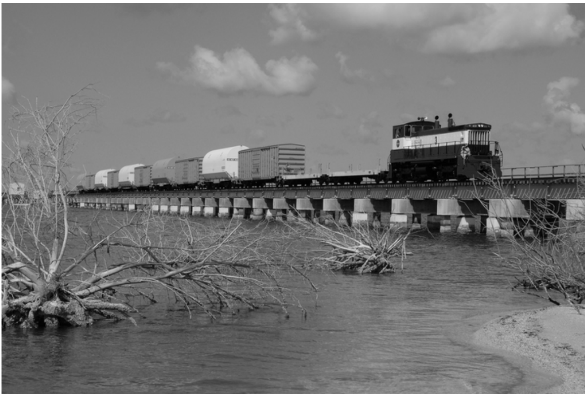
Figure A-17. Locomotive No. 3 carrying fueled SRM segments across the Jay Jay Bridge, March 20, 2009.
