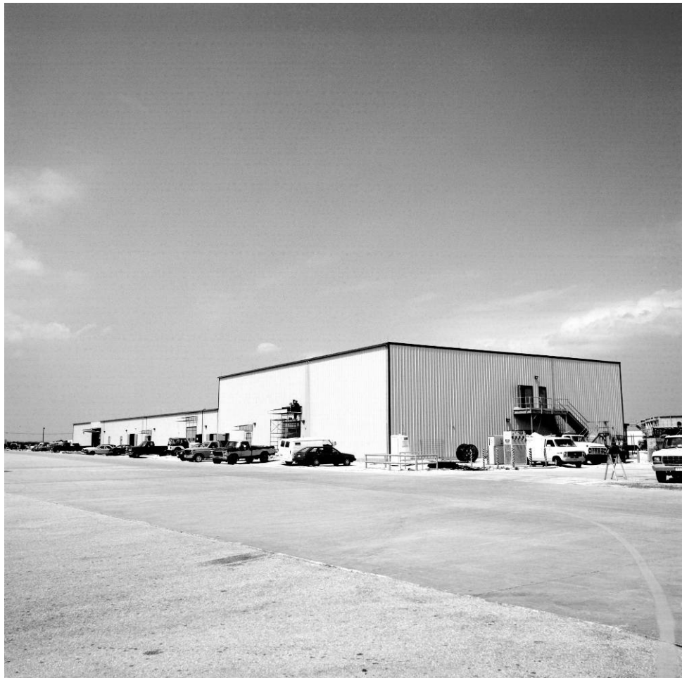
Figure A-1. View of TPSF while under construction at KSC, March 17, 1987. Source: John F. Kennedy Space Center Archives, KSC-387C-565.4.
