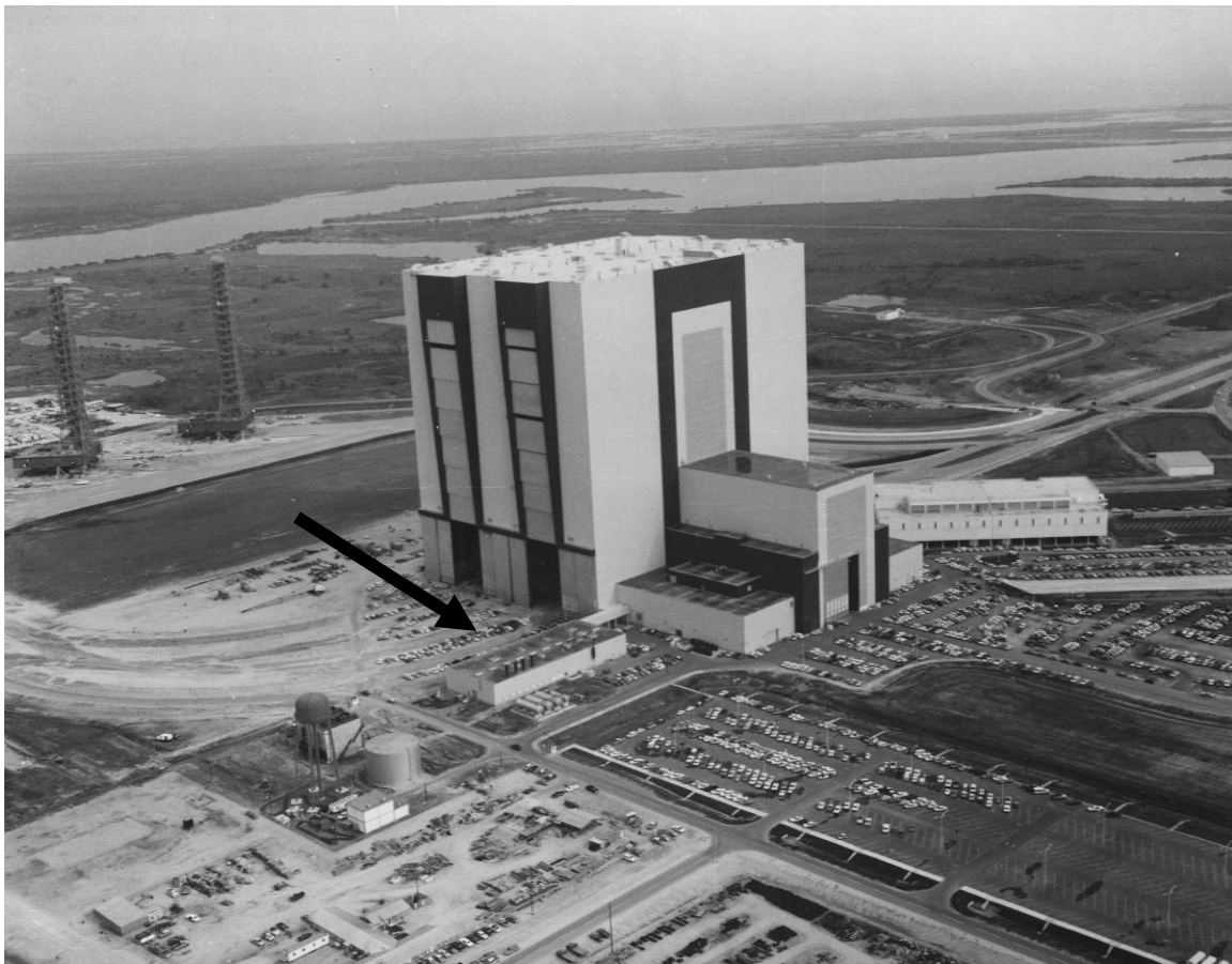
Figure B-4. View of VAB and VAB Utility Annex (denoted by arrow), facing northeast, January 7, 1966.
