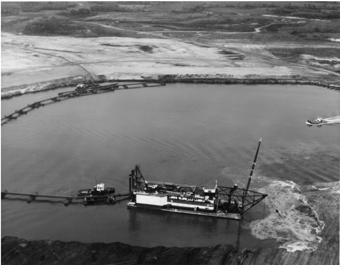
Figure D-3. Dredging of the Barge Terminal Facility, direction unknown, May 28, 1963. Source: John F. Kennedy Space Center Archives, LOC-63-5462.
