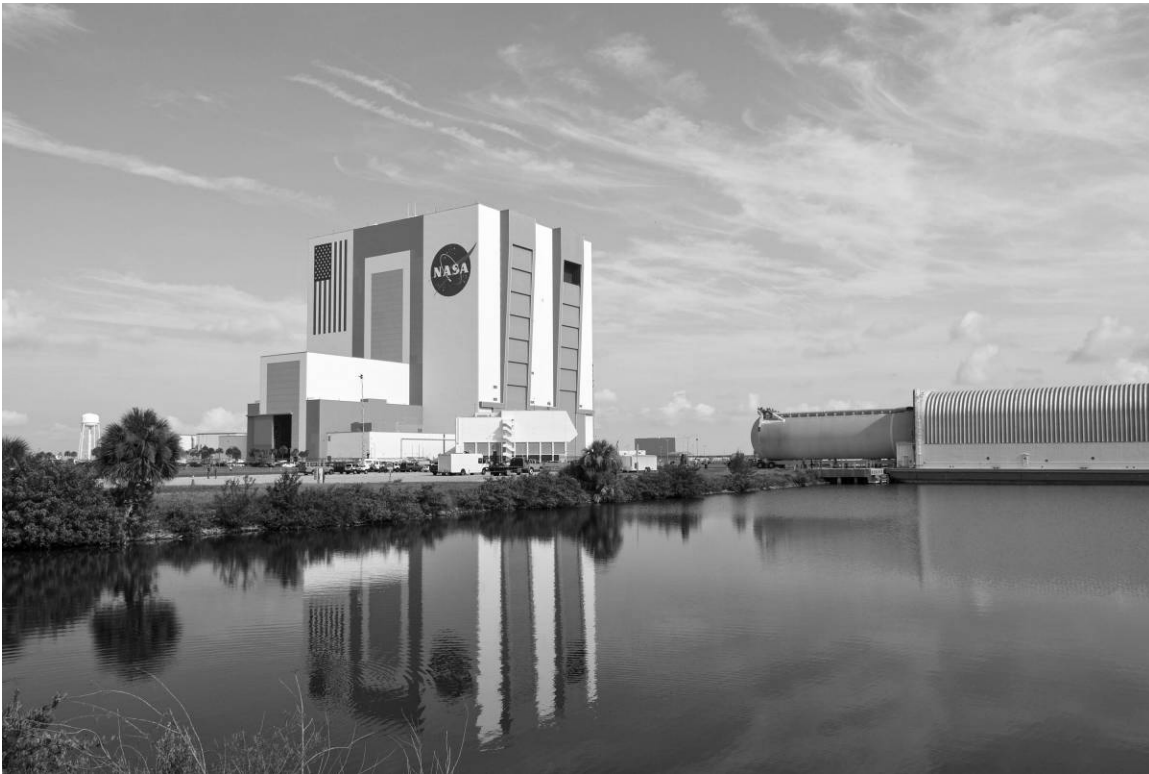
Figure D-12. The external tank for STS-135 being unloaded at the Barge Terminal Facility, facing northwest, July 14, 2010.
