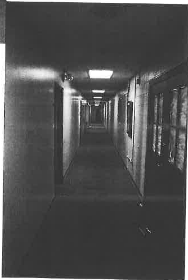
Hangar S, Second Floor Corridor Leading to Former Astronaut Quarters, View Northwest
