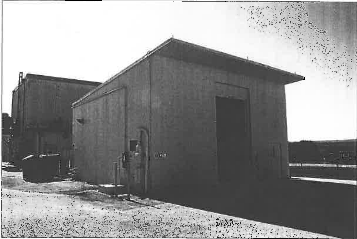
High Pressure Gas Building, Exterior
