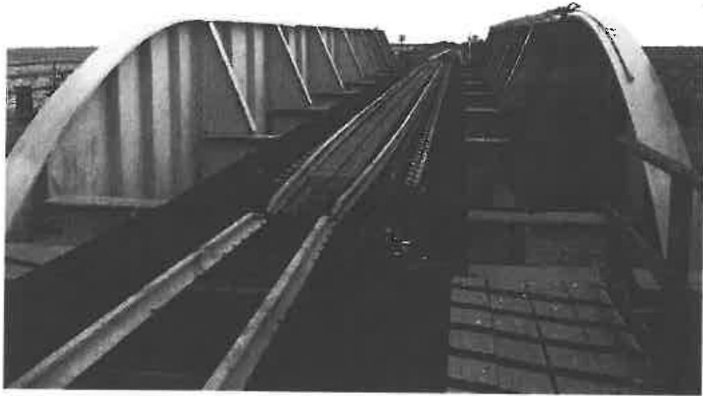
Jay Jay Bridge bascule lowered, facing east.
