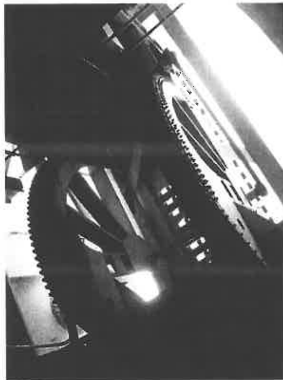
Jay Jay Bridge bascule gears, while bridge is being lowered.
