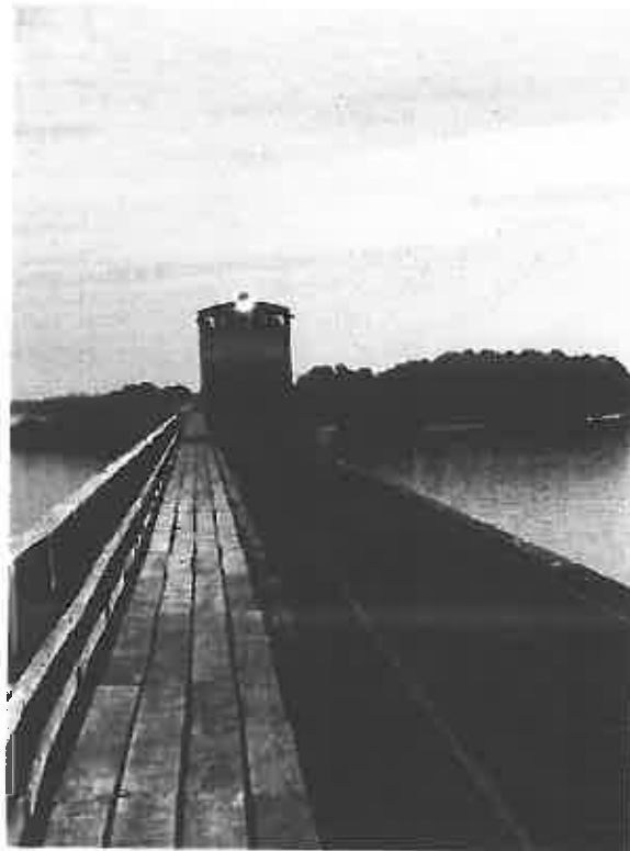
Locomotive 2 on Jay Jay Bridge facing east.
