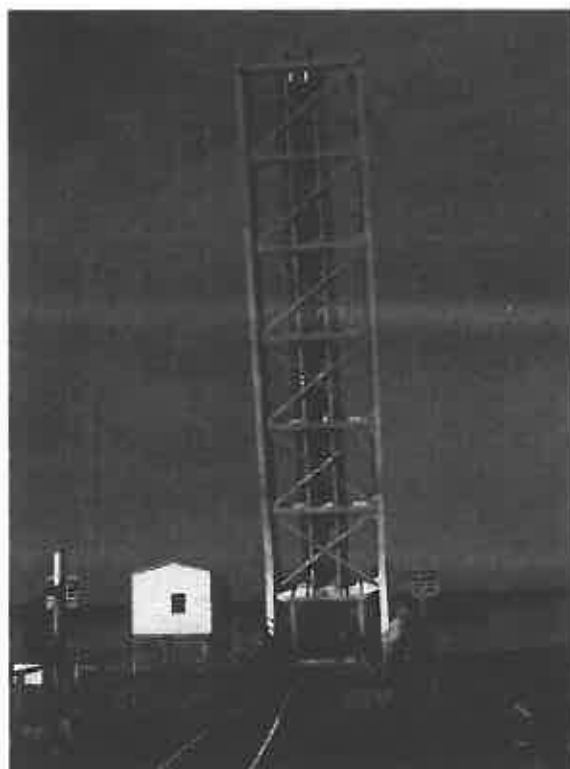
Jay Jay Bridge upright, after crewmember activated span, facing west.
