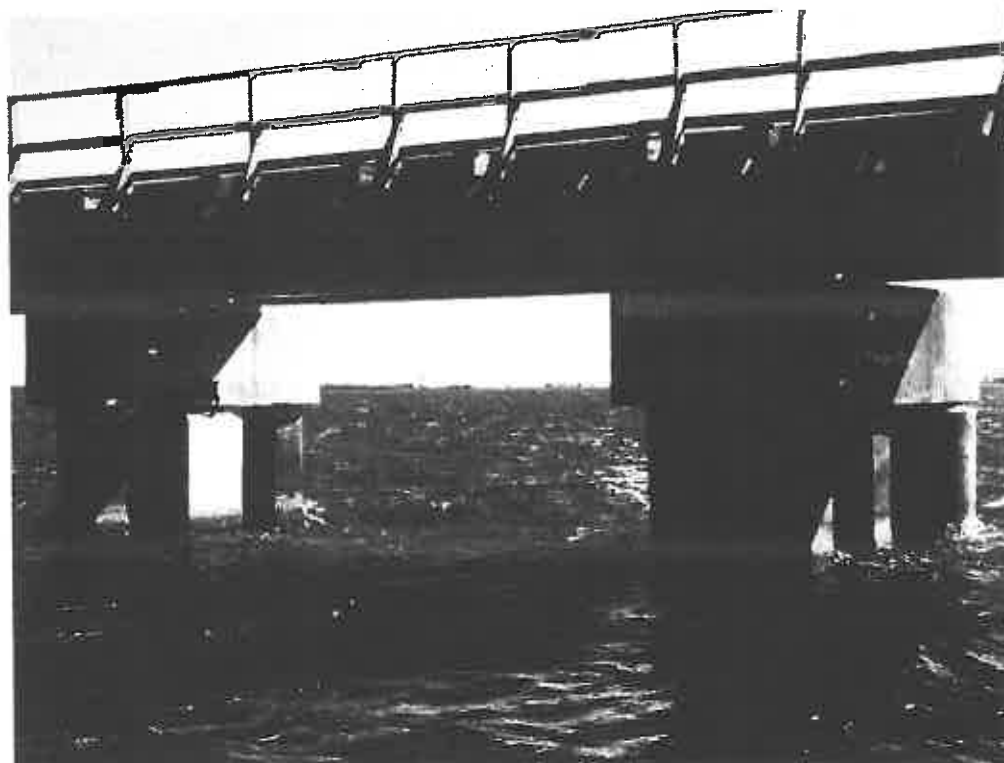
Jay Jay Bridge representative piles, facing southwest.
