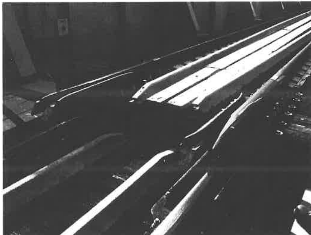
Jay Jay Bridge bascule tracks being lowered, facing northeast.
