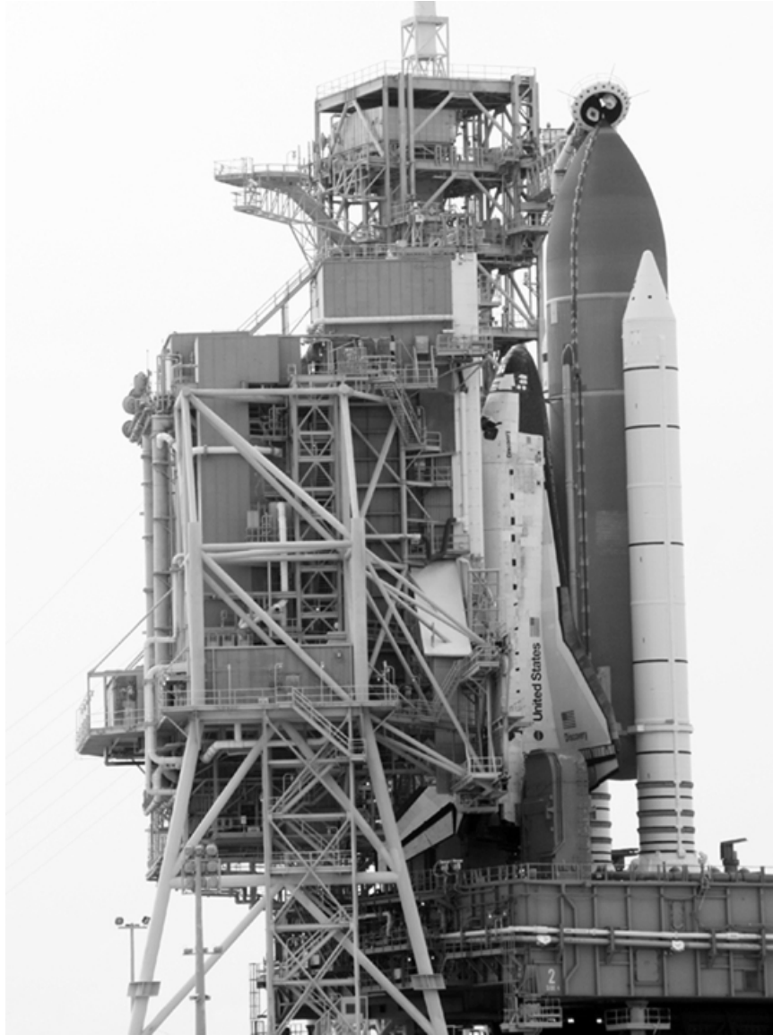
Photo B-15. View of RSS as it moves to its mated position around the orbiter, August 27, 2009. Source: John F. Kennedy Space Center, KSC-2009-4870, accessed via http://mediaarchive.ksc.nasa.gov/search.cfm .
