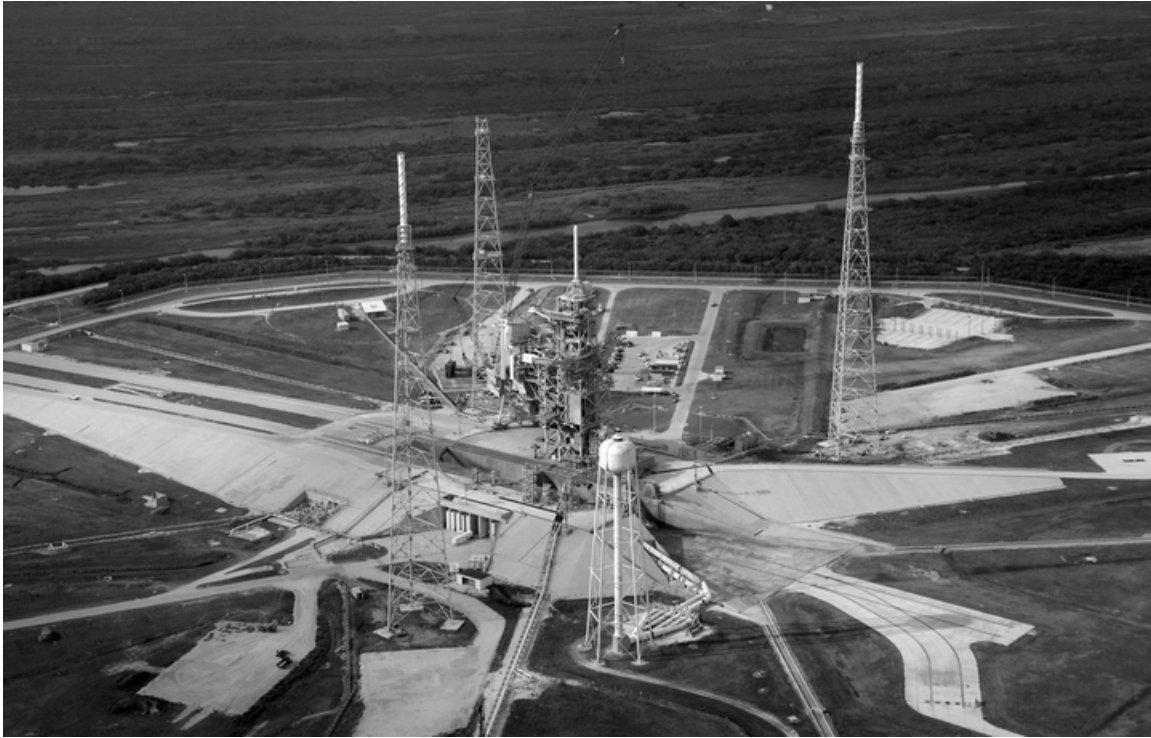
Photo C-4. LC39B during the installation of the new lightning protection system, February 12, 2009.
