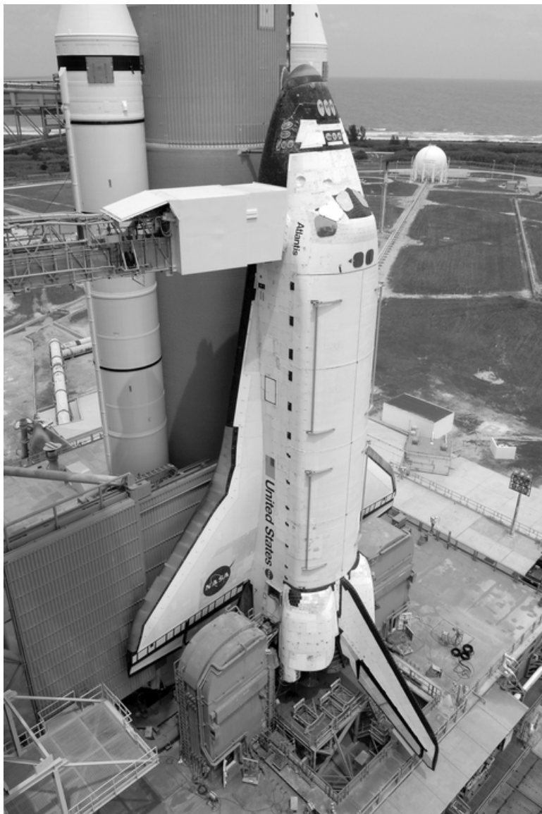
Photo B-14. View of various FSS access arms in their extended position, April 17, 2009. Source: John F. Kennedy Space Center, KSC-2009-2730, accessed via http://mediaarchive.ksc.nasa.gov/search.cfm .
