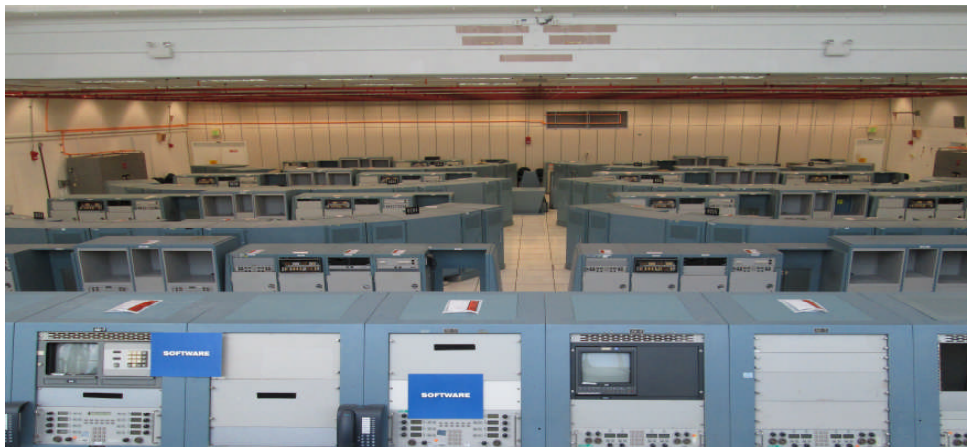
Overview of Firing Room 2, facing west.
