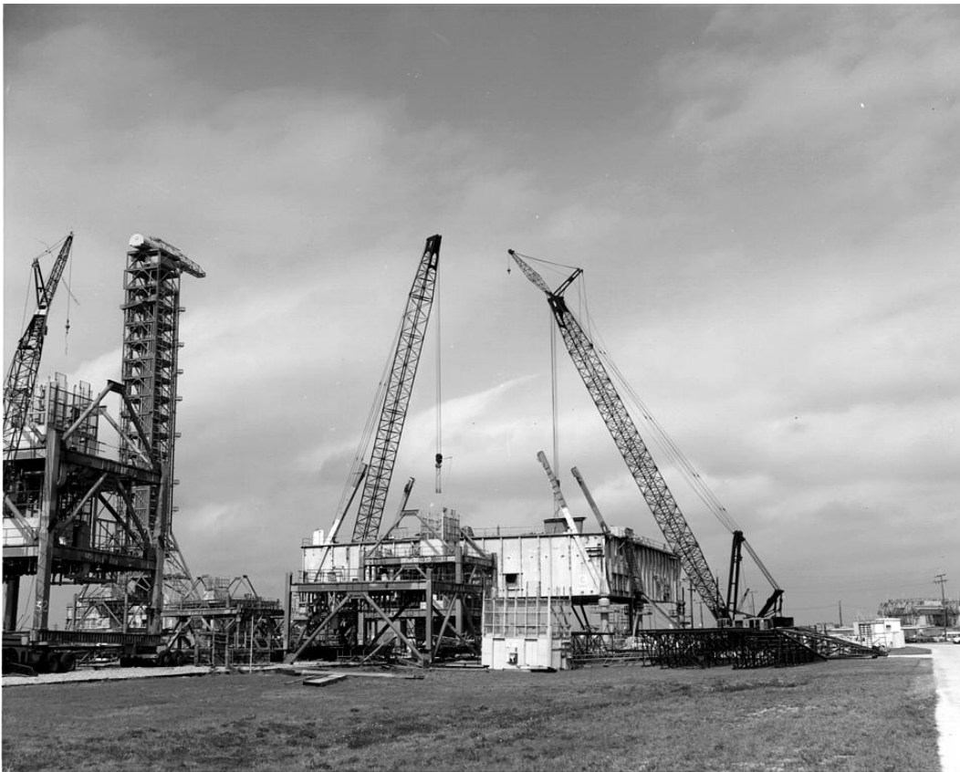
Figure A-3. Mobile Launcher No. 3 after removal of tower during modifications to become Mobile Launcher Platform No. 1, March 22, 1976.
