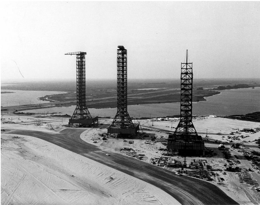
Figure A-1. Construction of mobile launchers, January 18, 1965.
