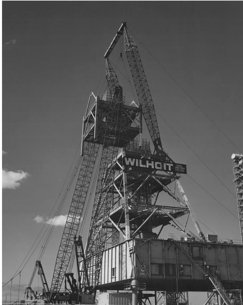
Figure A-2. Removal of the LUT from ML-3, March 2, 1976. Source: John F. Kennedy Space Center, KSC-76C-0715, accessed via NIX at http://nix.nasa.gov/ .
