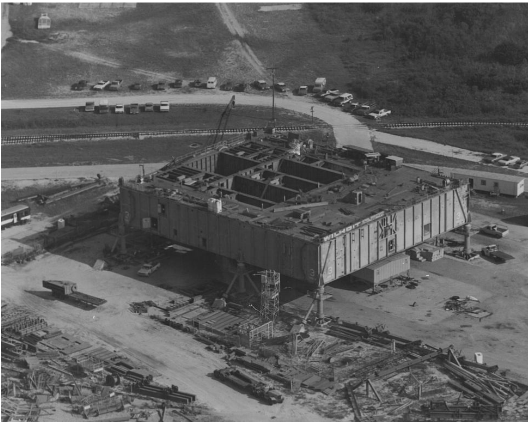
Figure A-4. Construction of Mobile Launcher Platform No. 1, September 24, 1976.
