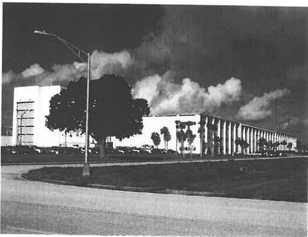
Photo 2. North and east elevations, facing southwest.
