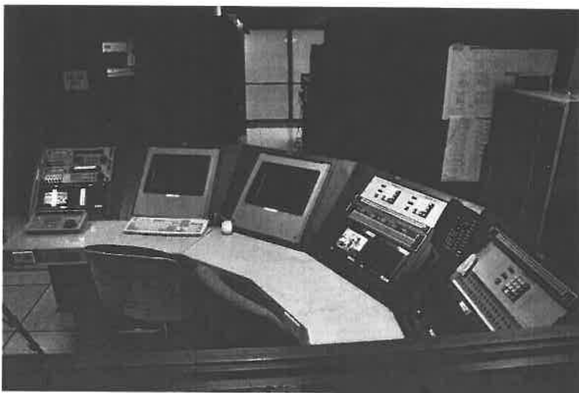
Photo 10. View of an original Apollo-era Acceptance Checkout Equipment console, facing south.
