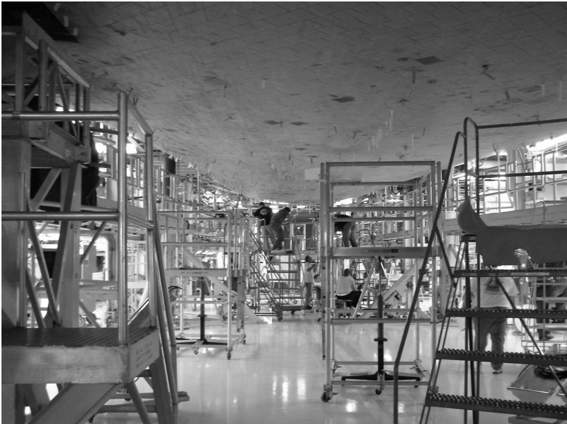
Figure A-7. Orbiter Processing Facility High Bay No. 3, orbiter underside with moveable platforms, looking north, July 31, 2006. Source: Archaeological Consultants, Inc.
