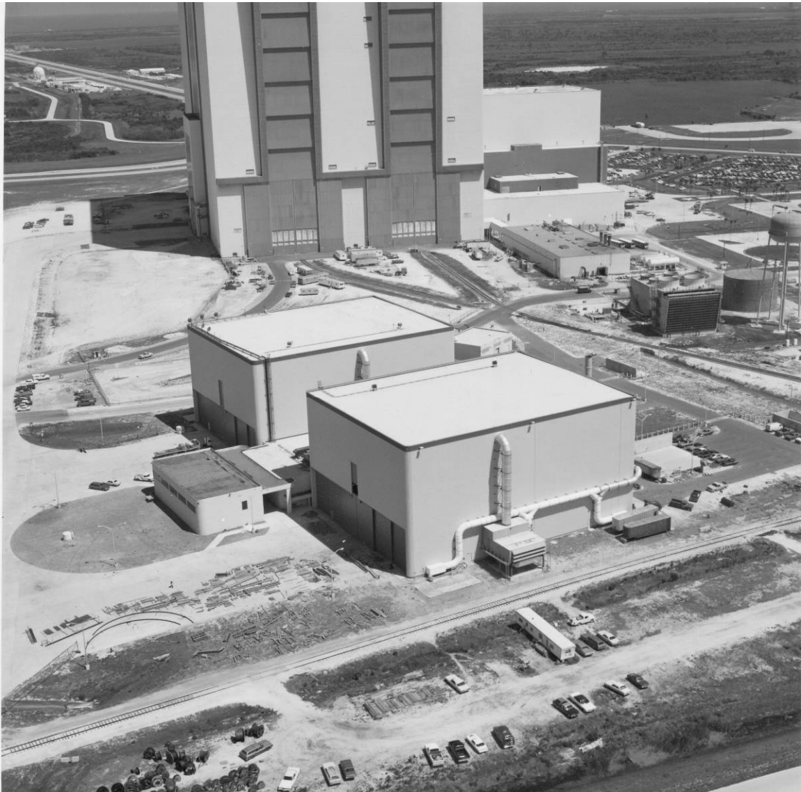
Figure B-6. View of original OPF, March 29, 1978. Source: John F. Kennedy Space Center Archives, 108-KSC-378C-202, Frame 35.
