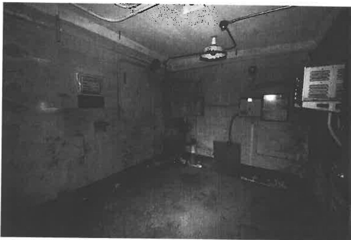
Photo 3. View of interior, facing northwest
