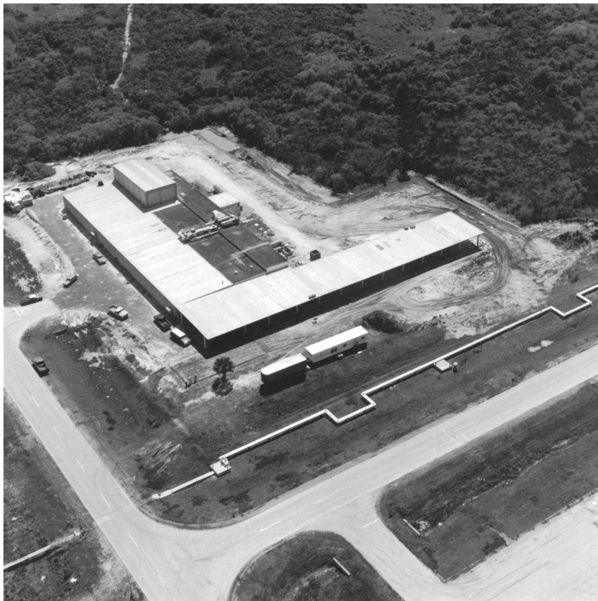
Aerial View of the Parachute Refurbishment Facility After Additions, View Southwest, 1978. (Source: KSC, Image 108-KSC-378C-201-1).
