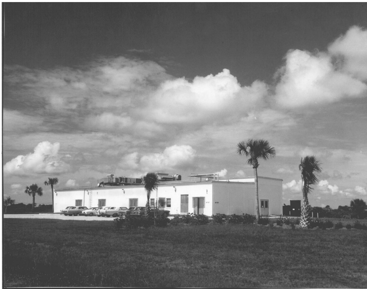
Photograph of the Original Parachute Refurbishment Facility Before Additions, View Southwest. (Source: KSC, Image 105-KSC- 66C-5579).
