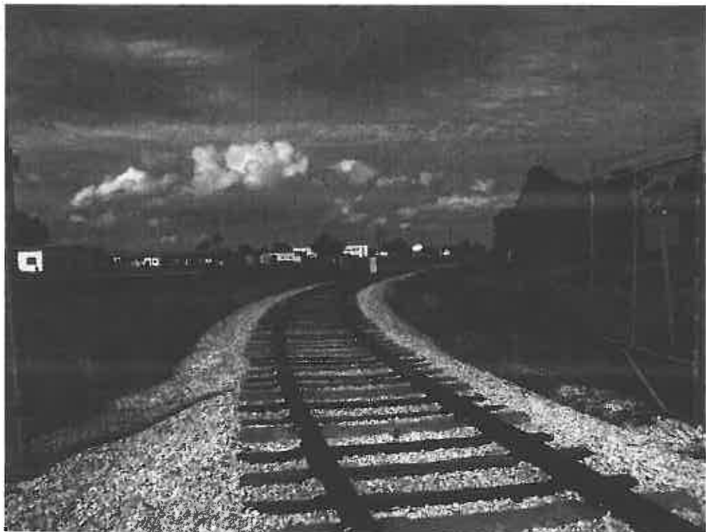
Track within the KSC Industrial Area, facing northwest
