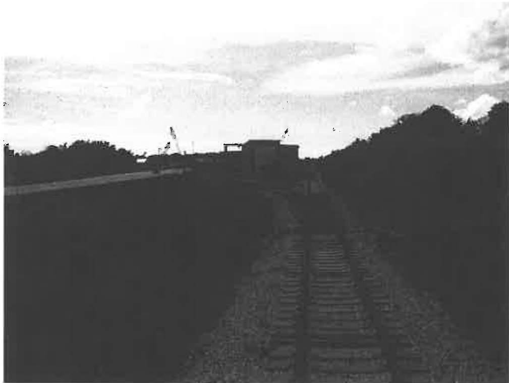
Track near the Locomotive Maintenance Facility, facing south
