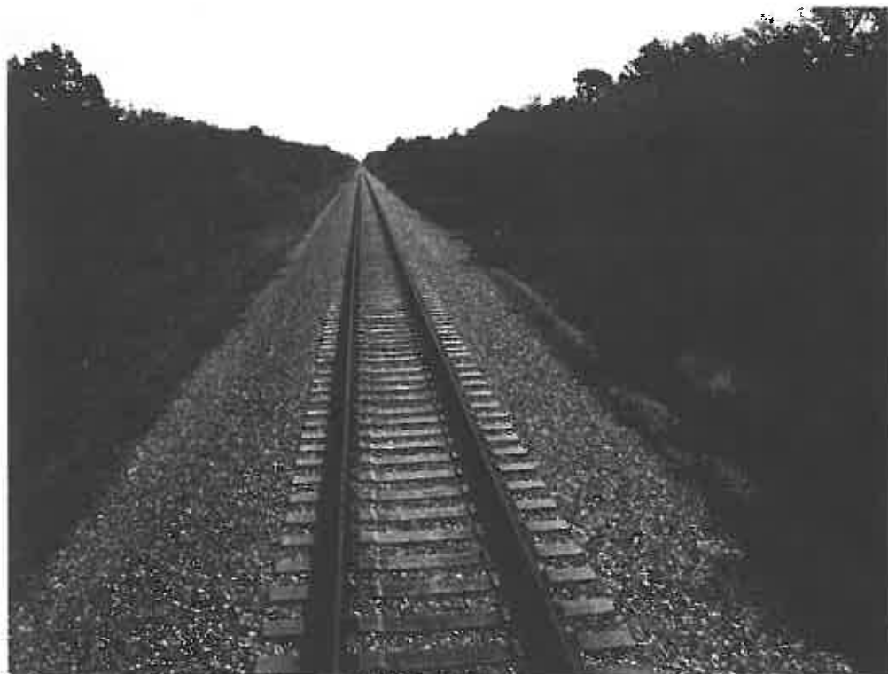
Track between Jay Jay Yard and Wilson's Corner, facing east
