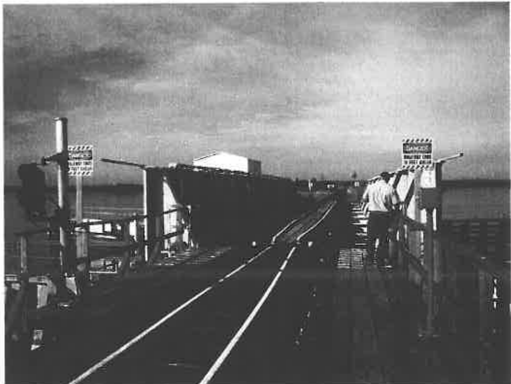
Track over Jay Jay Bridge, facing west
